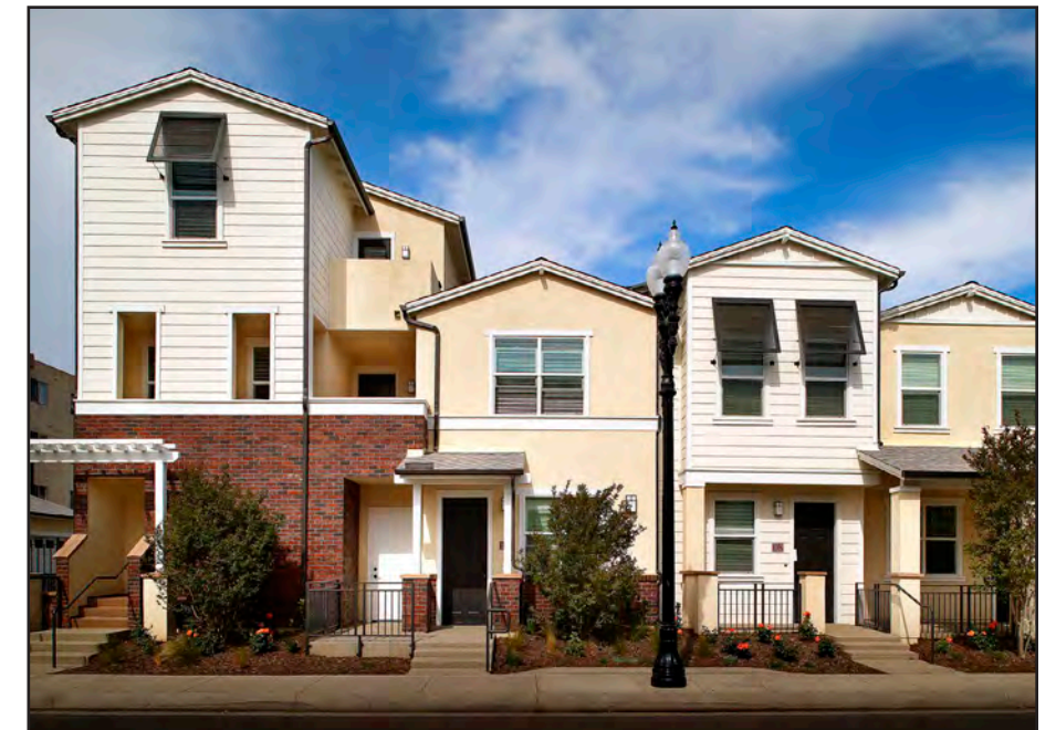
Photo 12. View of typical urban neighborhood.
