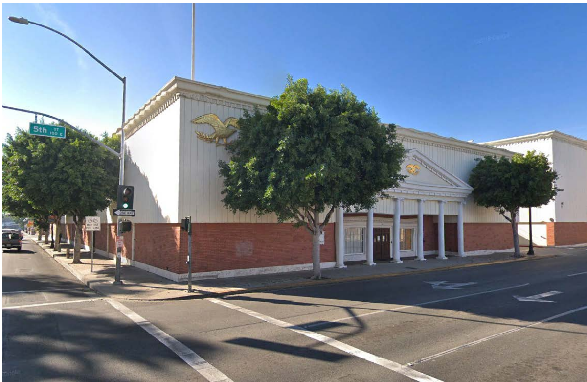
Figure 3.1-3 Southwest View of Parcel 1 from Fifth Street and North Bush Street
