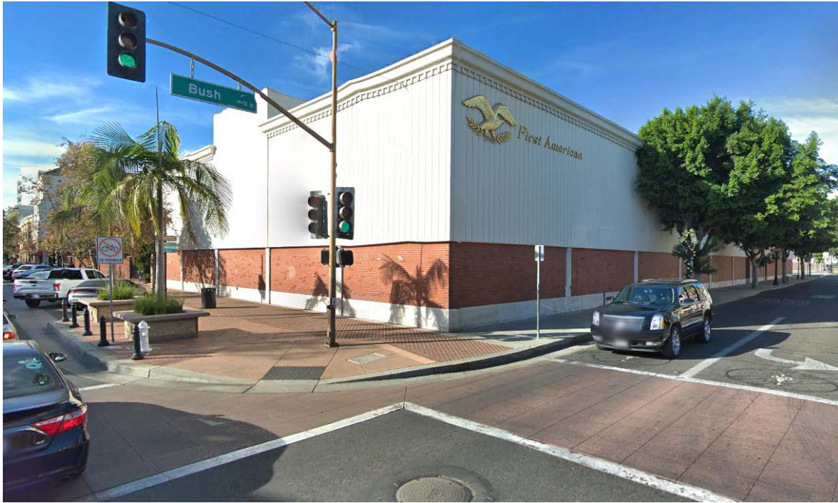
Figure 3.1-4 Northwest View of Parcel 1 from Fourth Street and North Bush Street
