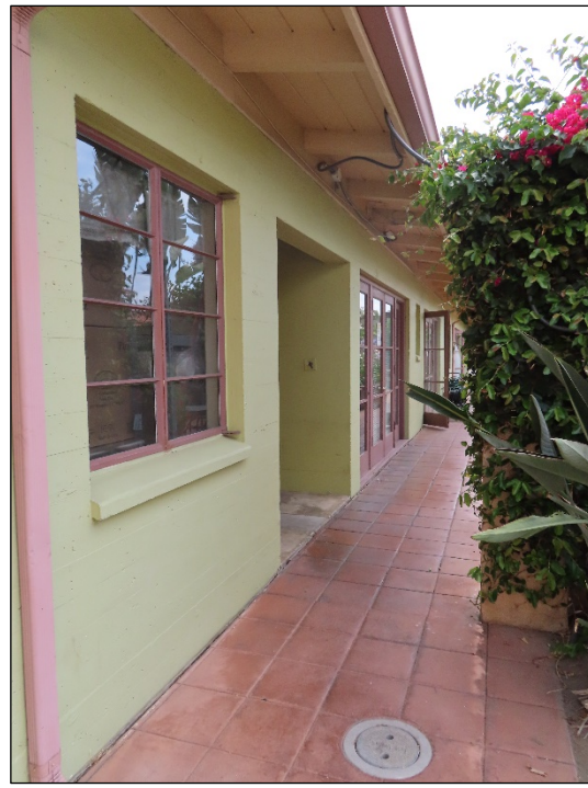
View west of the north façade.
