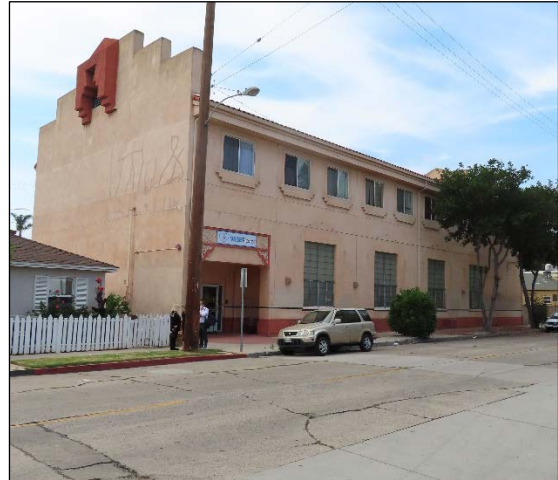
View northwest of the east and south façades from North Sycamore Street.
