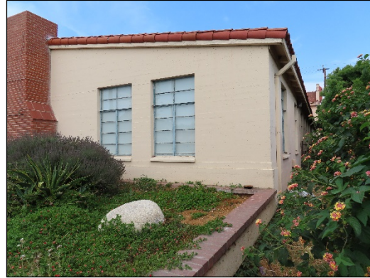
View east of the west and south façades.
