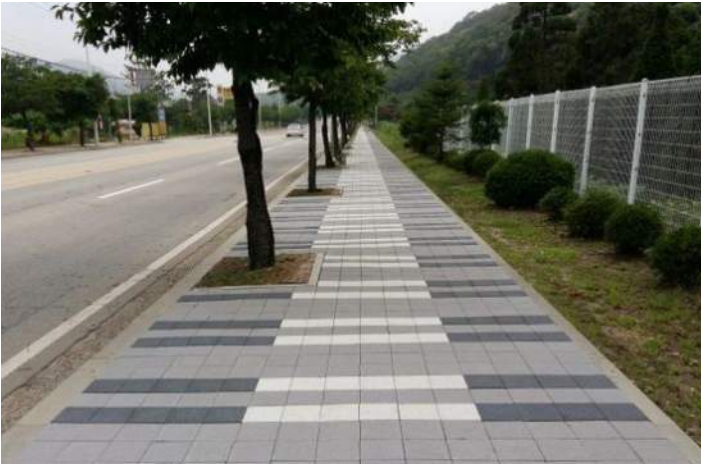
A Enhanced Paving
