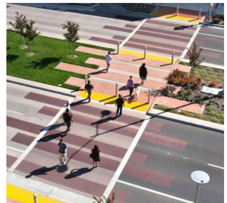
Decorative Crosswalk Paving
