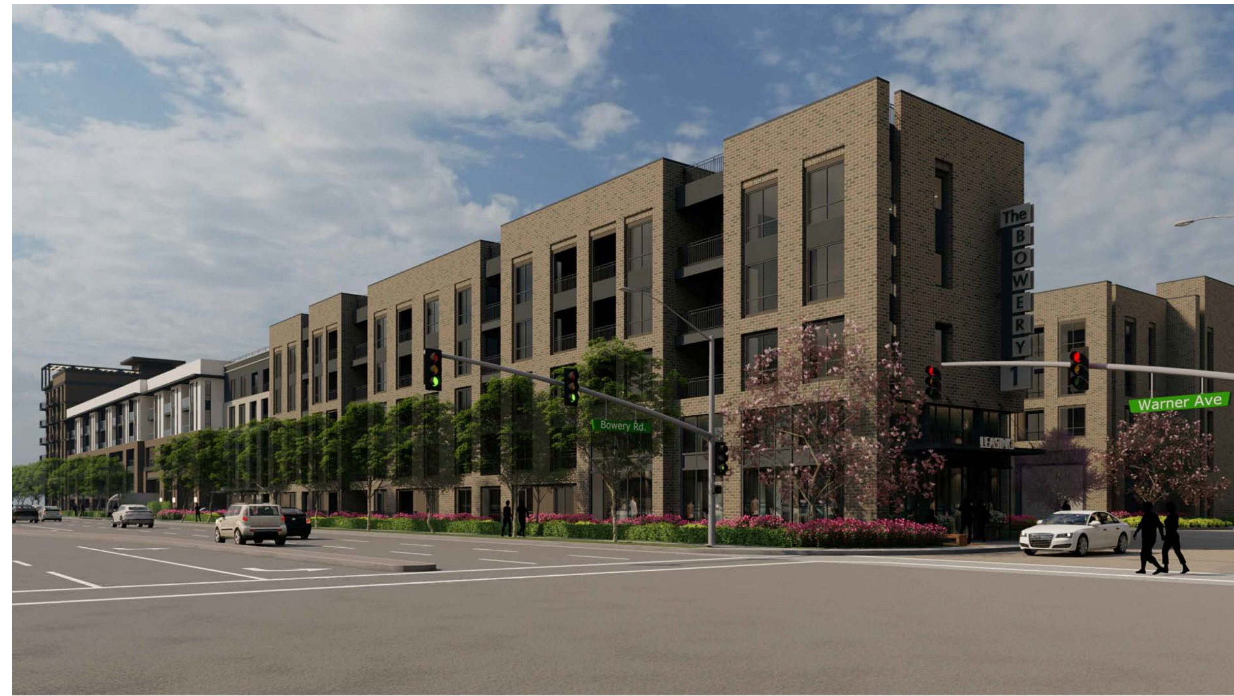
BLDG.'A' LOOKING EAST AT LEASING OFFICE 2
