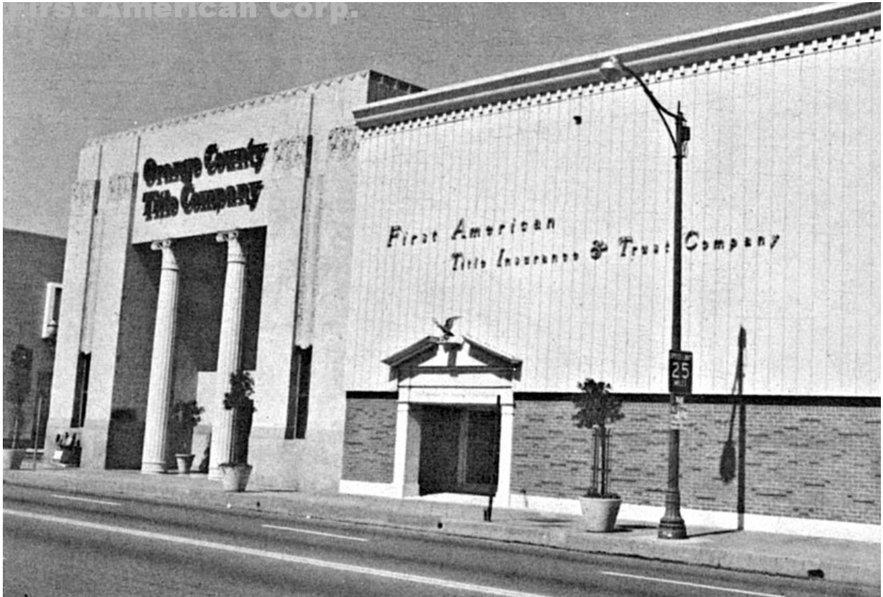
View of First American Title Building, Main Street elevation looking north. photo ca 1963
