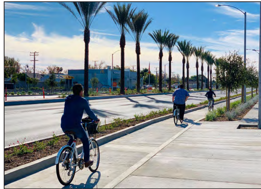
Photo 8. View of bike lanes on Bristol Street Corridor.
