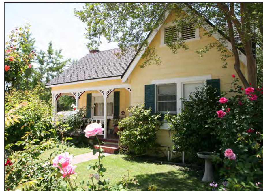
Photo 11. View of historic home in Wilshire Square.
