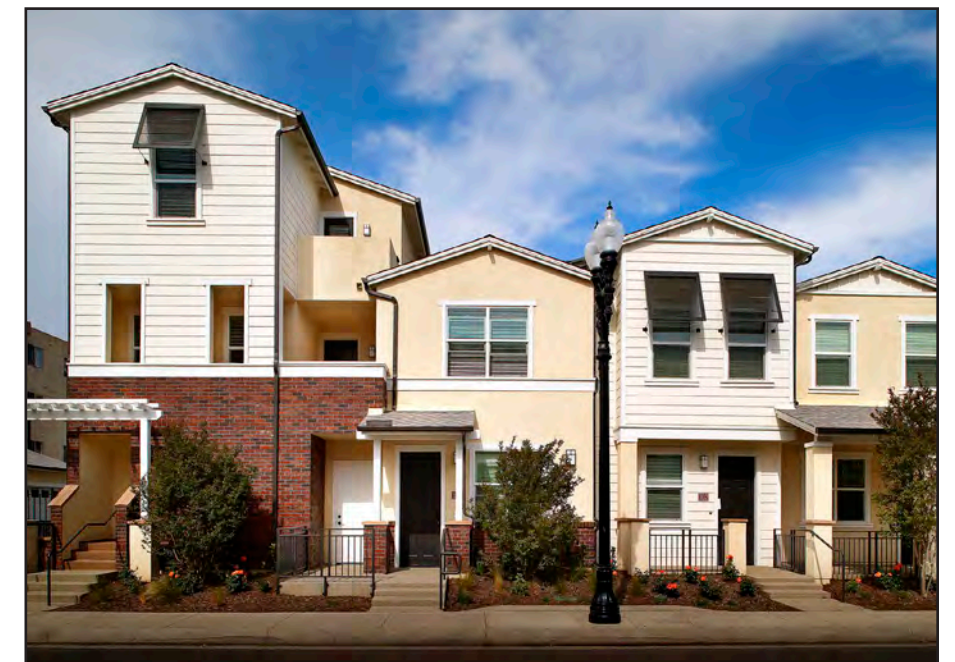
Photo 12. View of typical urban neighborhood.
