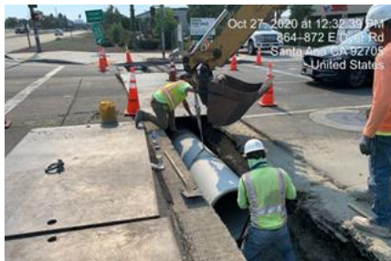
Dyer Road Stormdrain Repair
