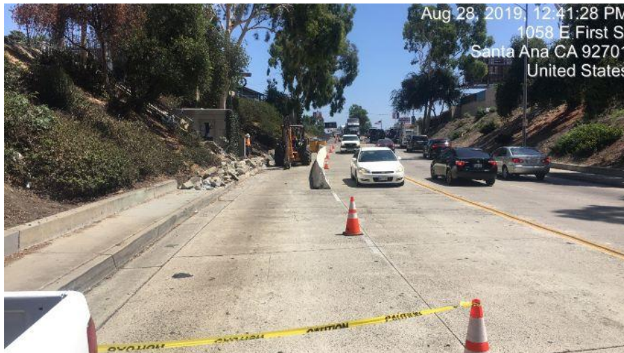
First Street Lift Station
