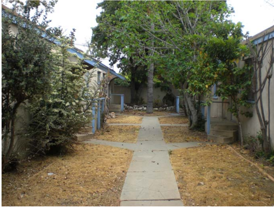
Picture 3: View between two (2) of the multi-family residential buildings at 611 North Minter Street.
