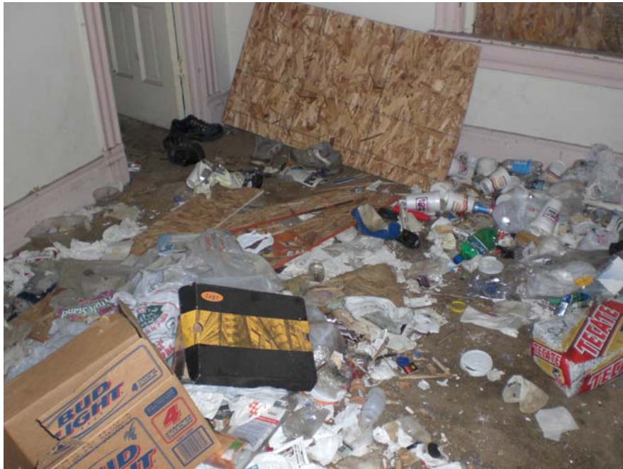
Picture 10: View of household trash and debris inside the 507 Mortimer Street structure.
