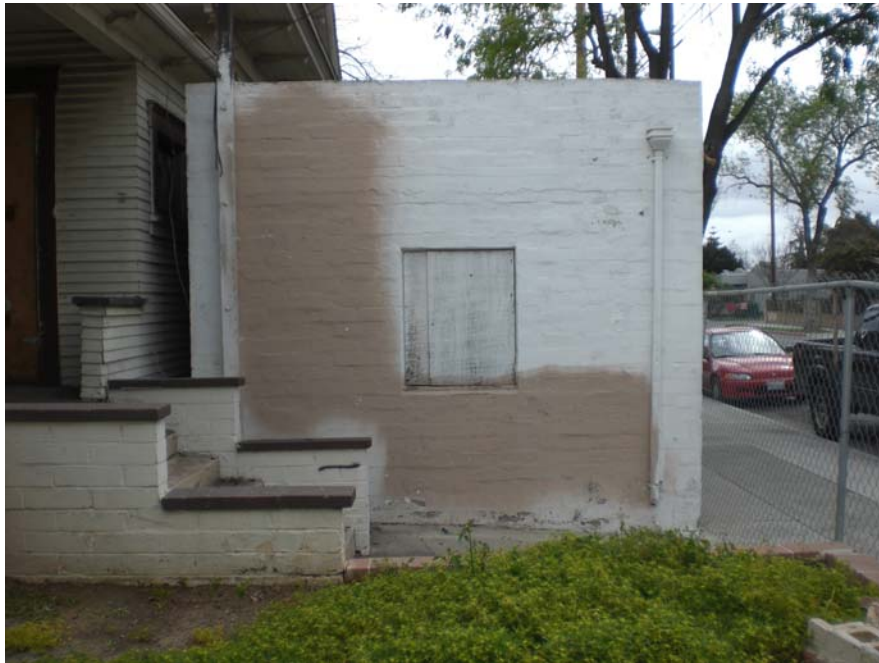
Picture 2: View of historic store structure at 505 East 5 th Street.
