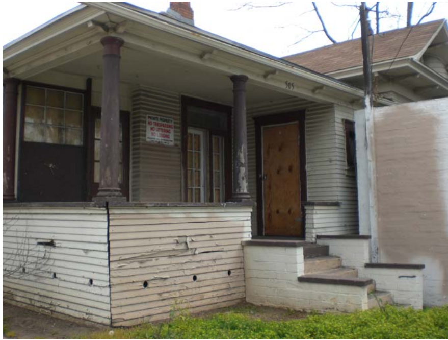
Picture 1: View of 505 East 5 th Street structure (main house).
