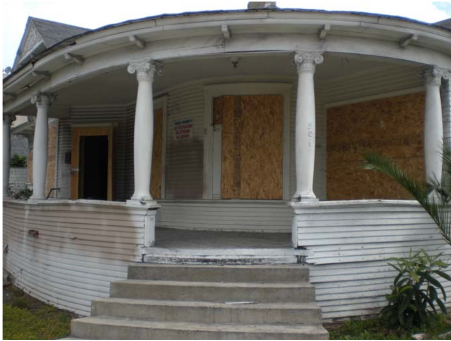
Picture 5: View of the 501 East 5 th Street main house (two-residential units).
