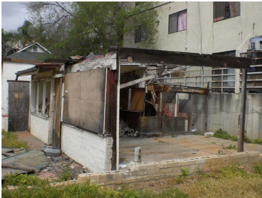
Picture 4: View of the dilapidated shed on the northern portion of the Property.
