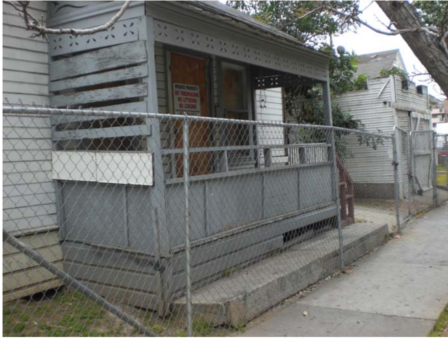
Picture 7: View of 507 Mortimer Street structure.
