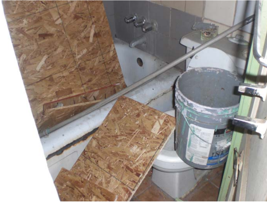
Picture 7: View of 5-gallon paint bucket inside 610/612 East 5 th Street structure.
