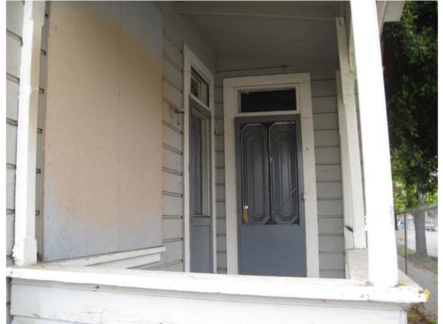
View of entrance to 505-507 North Minter Street.
