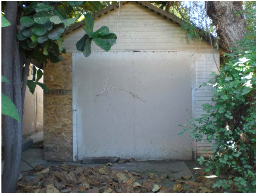
Picture 2: View of the shed at 714 E. 6 th Street.
