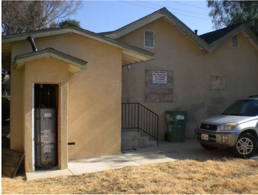
Picture 3: View of the rear of the main building at 710 E. 6 th Street.
