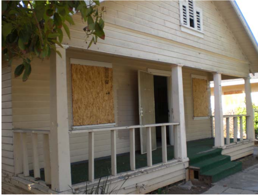
Picture 1: View of 714 E. 6 th Street main building.
