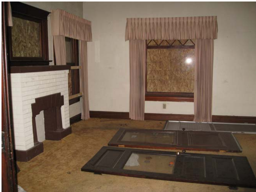
View of the interior of the 615-617 East 5 th Street dwelling.
