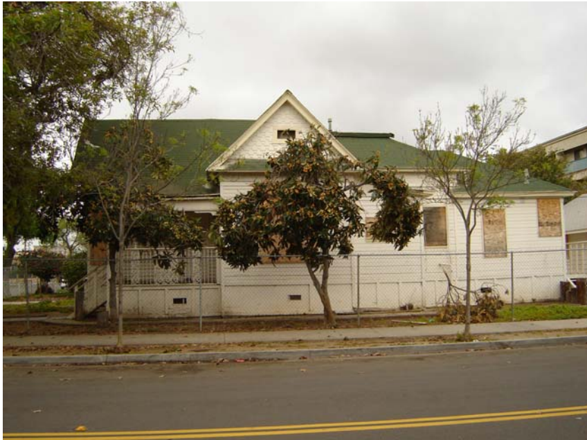
View of the 621 East 5 th Street duplex.
