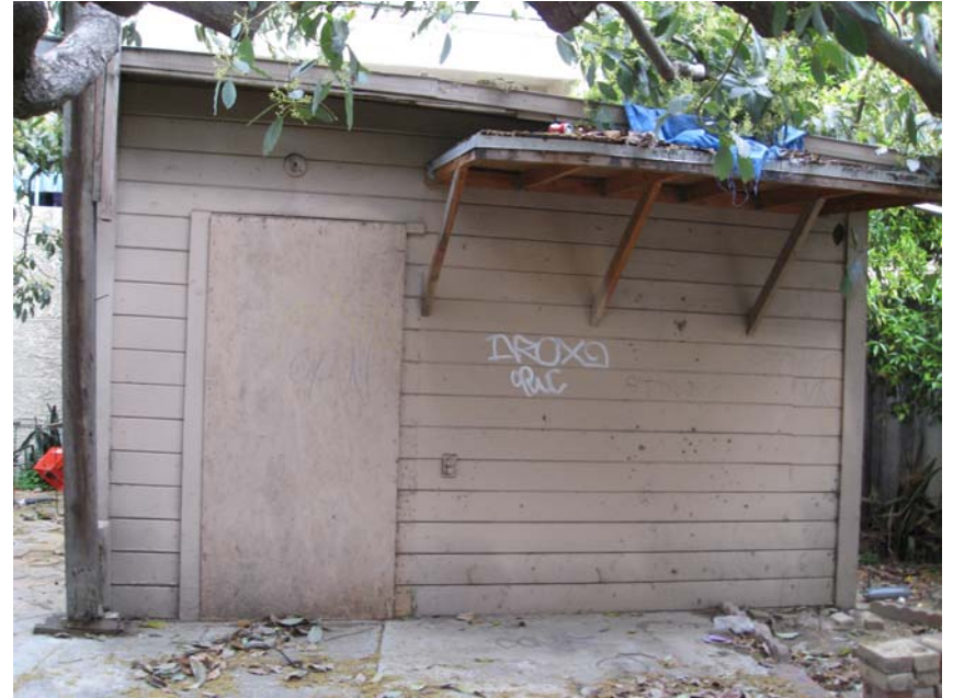
View of the garage on the northwestern portion of the Property.
