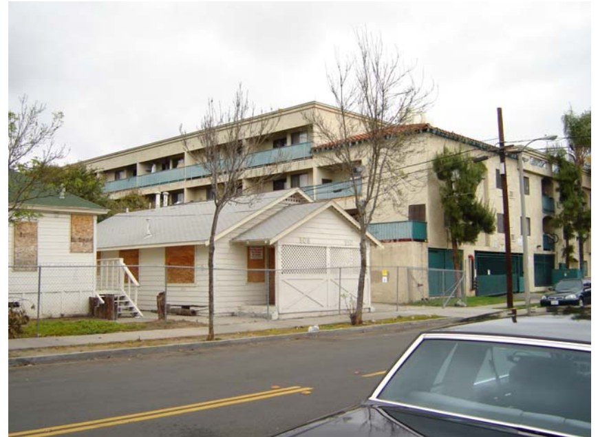
View of the 508-510 North Porter Street duplex.
