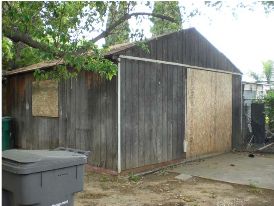
Picture 2: View of the onsite detached garage.
