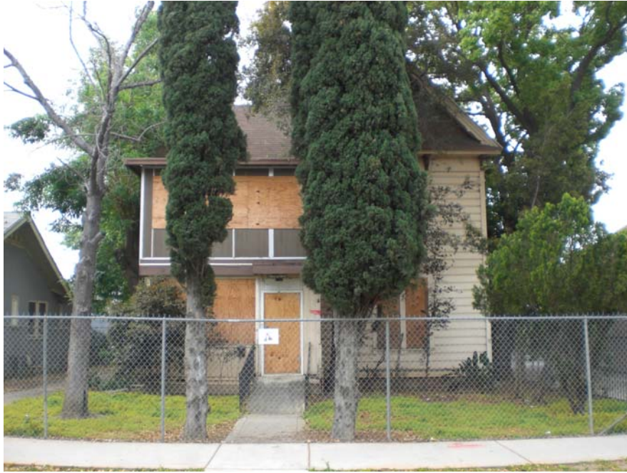
Picture 1: View of 712 East 5 th Street residential structure.
