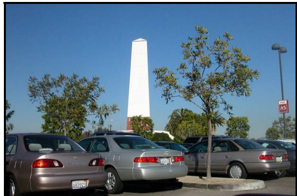
Figure 10-45: Example of a cell tower concealed within an obelisk
