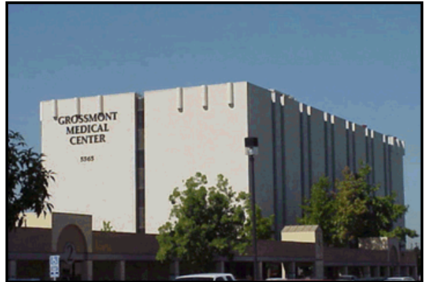
Figure 10-47: Example of a wall-mounted cellular site
