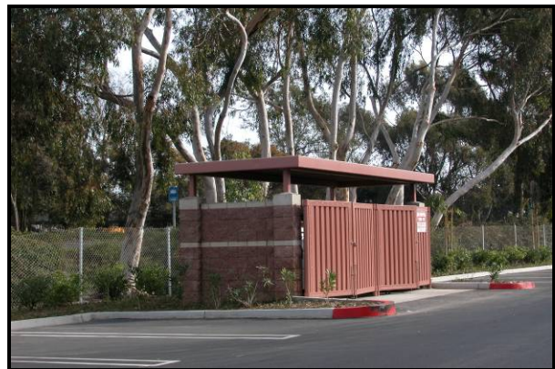
Figure 10-43: Refuse enclosures should be designed to minimize odors to adjacent residential and non-residential uses
