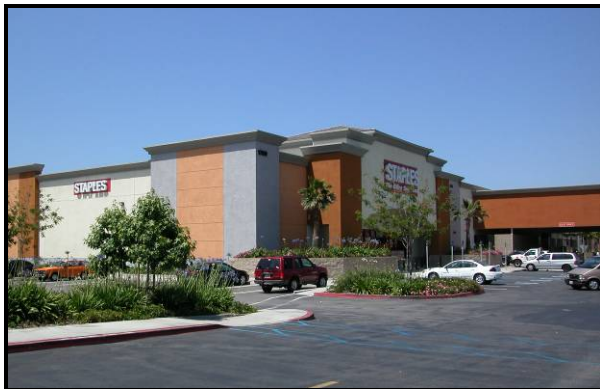
Figure 10-33: Example of big box retail in Santa Ana
