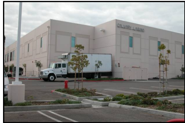
Figure 11-29b: Loading/unloading facilities should be designed in consideration of the scale of transport vehicle
