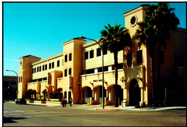
Figure 12-2: The ground floor should be used for retail or other appropriate use and be articulated in a manner to lessen the appearance or mass and bulk
