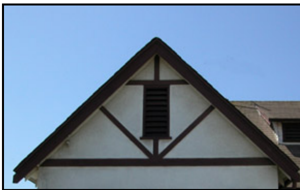
Figure 13-31: Vent replacement should match the original design
