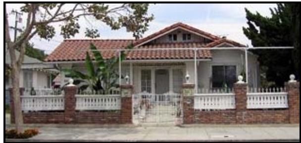
Figure 13-50: Example of inappropriate fence
