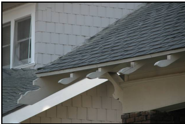
Figure 13-25: Flat wood shingles are typical of the Victorian and Craftsman styles
