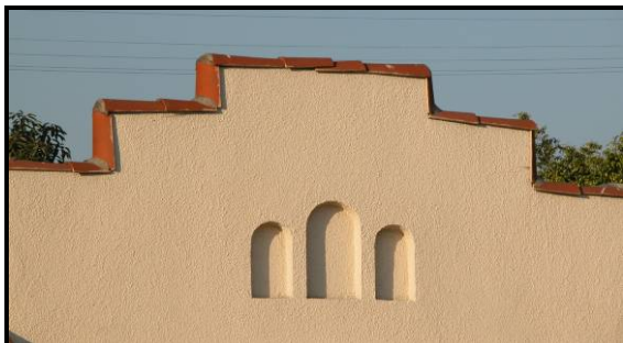
Figure 13-13: Example of exterior plaster (stucco)
