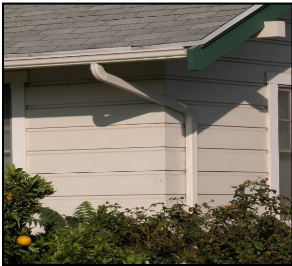
Figure 13-8: Example of clapboard
