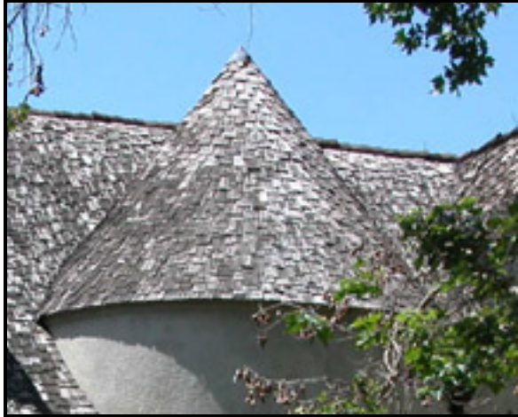
Figure 13-24: Thatched roofing is typical of the Tudor style.
