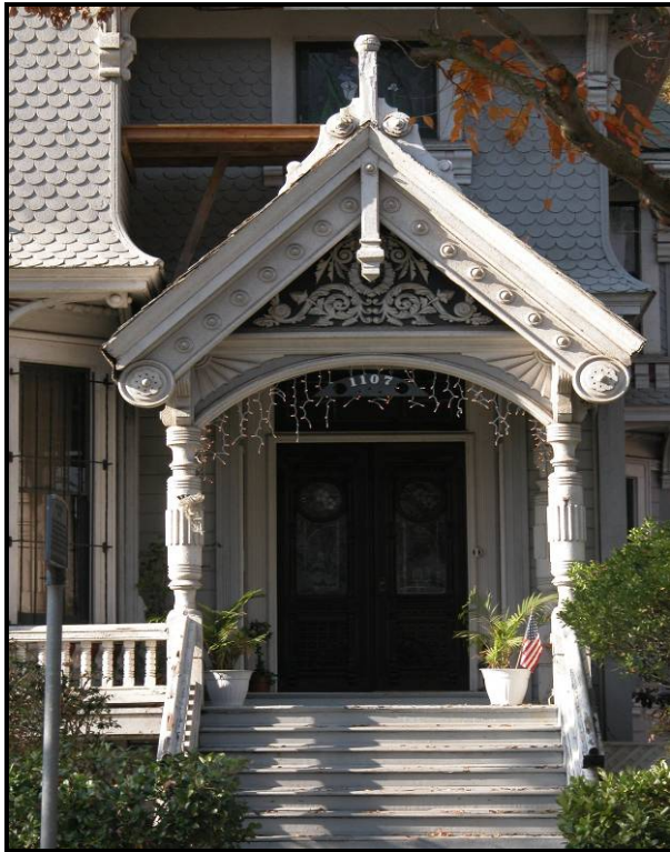
Figure 13-15: Example of typical Victorian-era porch detail
