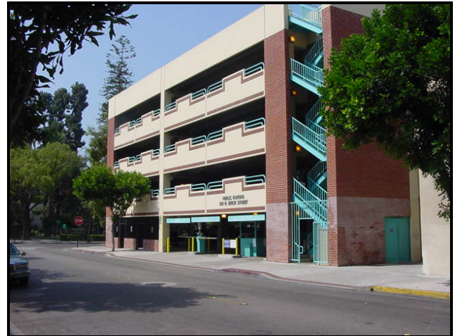
Figure 5-1: Example of an open staircase in a parking structure
