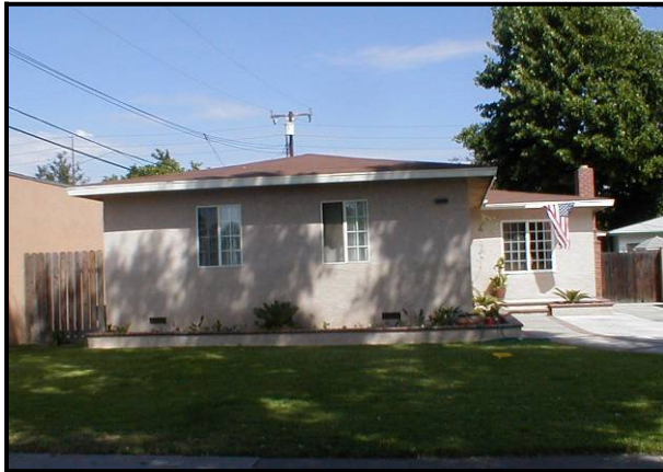
Figure 6-36: Inappropriate window change out
