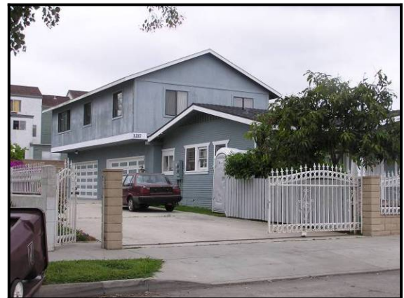
Figure 6-14b: Addition is not in proportion to the scale of the original building
