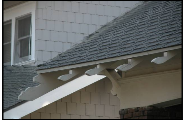
Figure 6-19a: Flat wood shingles are typical of the Victorian and Craftsman styles
