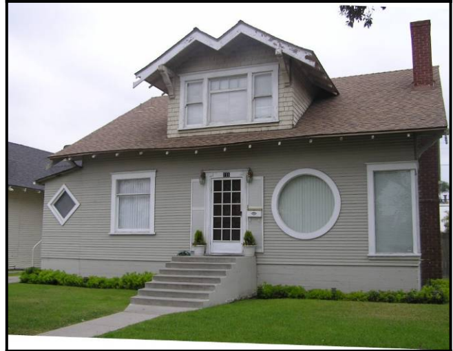
Figure 6-34: Avoid windows that are not complementary to the style
