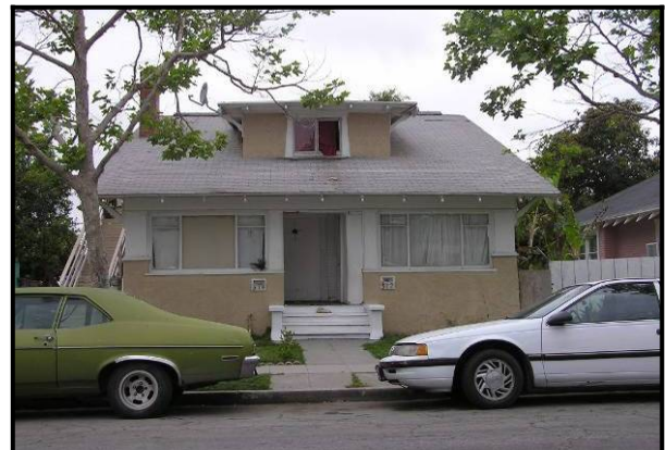
Figure 6-27b: Inappropriate porch enclosure
