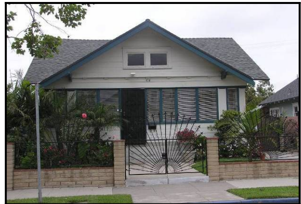
Figure 6-27a: Inappropriate porch enclosure
