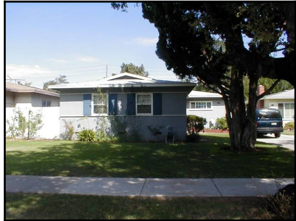
Figure 6-37: Appropriate window replacement includes preservation of architectural features
