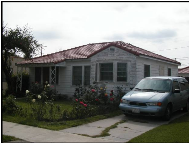
Figure 6-29: Avoid introducing materials that are not complementary to the building style. Red roof tiles are not complementary with cottage style.
