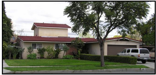
Figure 6-14a: Addition is not in proportion to the scale of the original building
