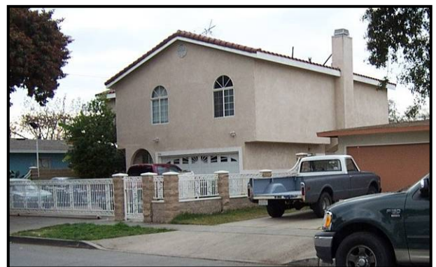
Figure 6-9: Inappropriate scale and mass of the second story
