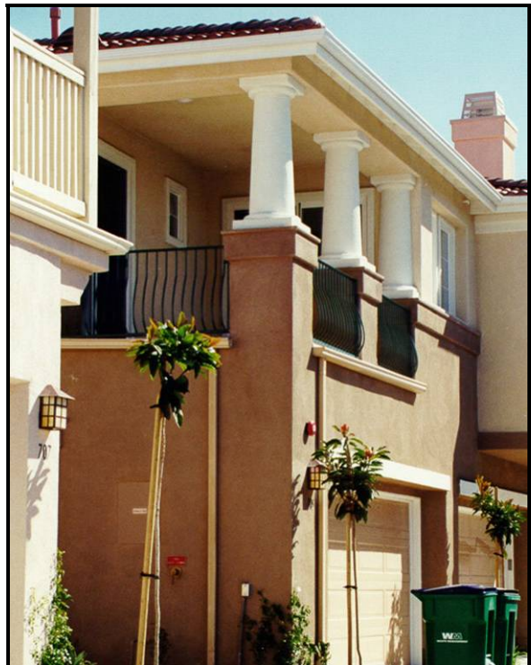
Figure 7-8: Break up large wall masses through the use of balconies and porches
