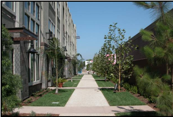
Figure 7-51: Plantings should soften the area between the property line and the buildings
