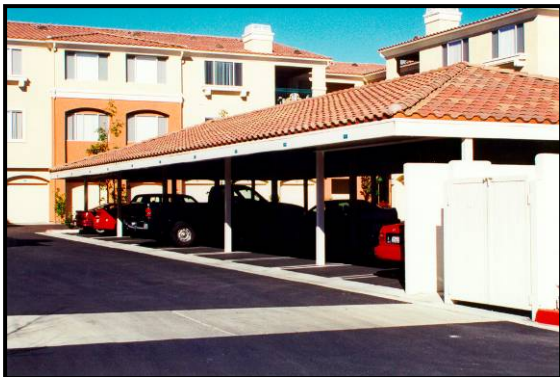
Figure 7-26: Parking facilities should complement the design of the development’s architecture
