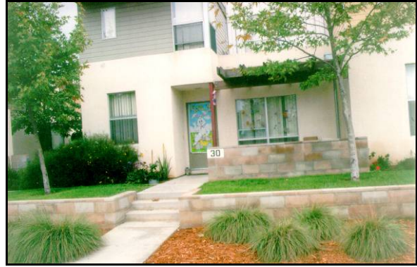
Figure 7-53: Low retaining walls in the front yard
