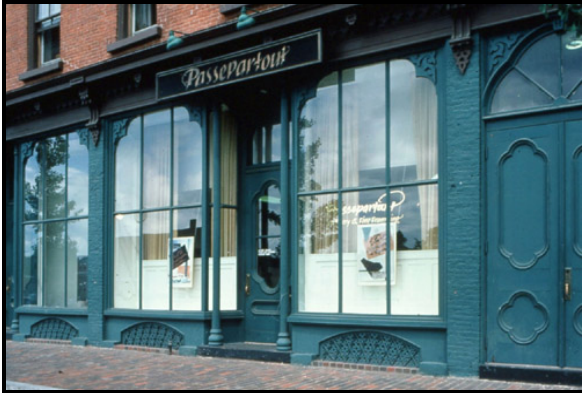
Figure 8-17: Preserve architectural metals and historic colors or finishes
