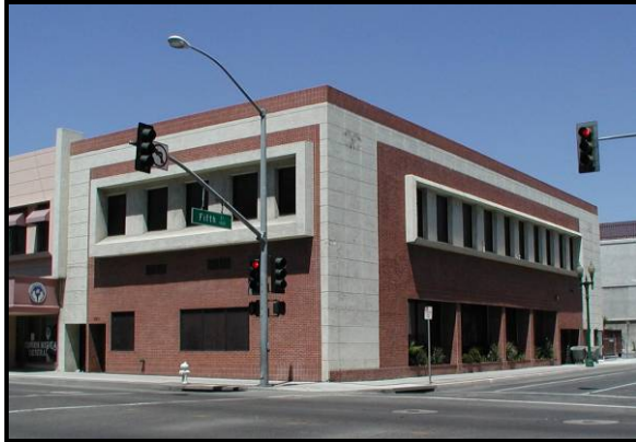
Figure 8-3c: Numerous alterations to this 1929 building has left it with little or no visible historic fabric
