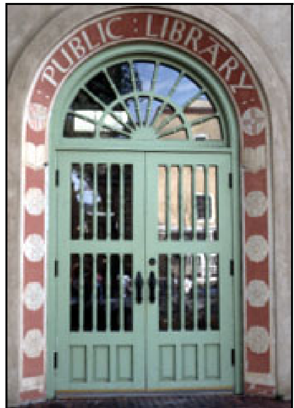
Figure 8-9a: Example of original door style
