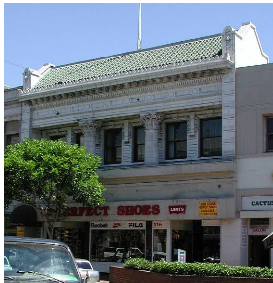
Figure 8-3b: Modified Orange County Savings and Trust Co. Building.
