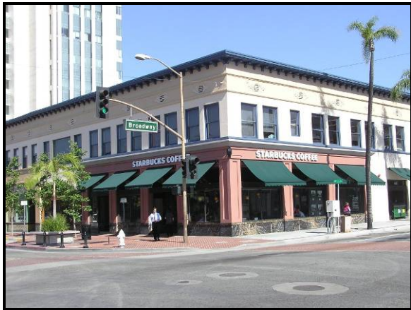
Figure 8-19b: Example of appropriate retractable awnings
