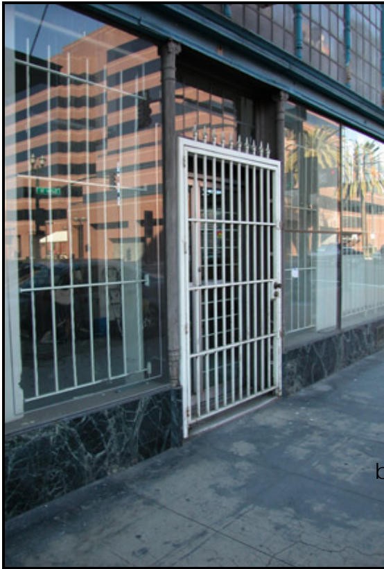
Figure 8-9b: Example of inappropriate use of security door
