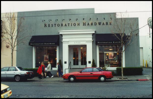
Figure 9-14: Building entries should be easily identified
