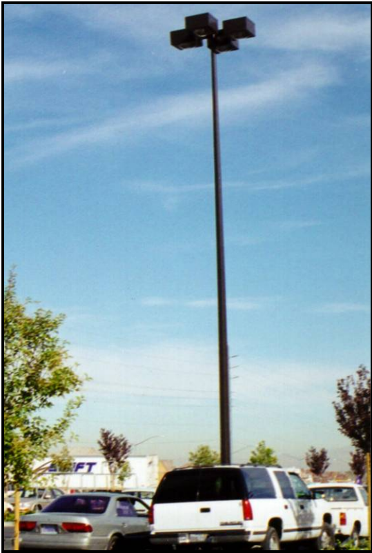
Figure 9-46: Parking lot lighting fixtures should be appropriately scaled. Avoid excessive fixture heights.
