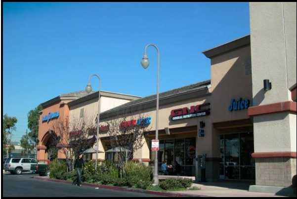
Figure 9-1: Example of commercial development in Santa Ana
