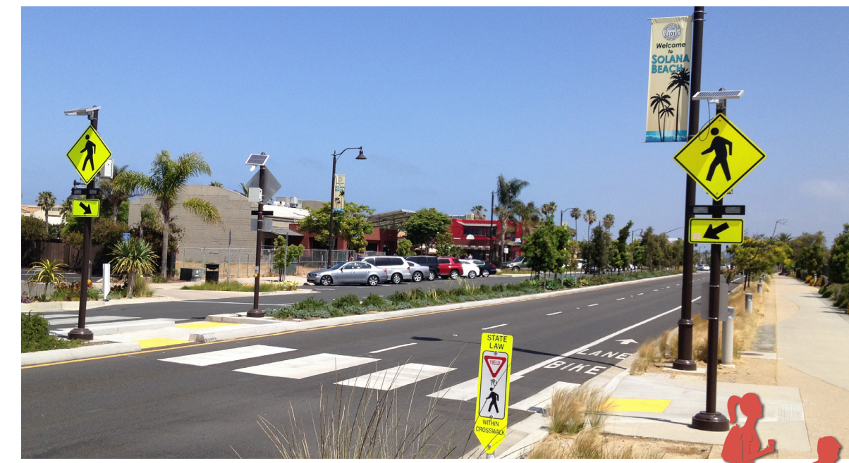
Rectangular Rapid Flashing Beacon
