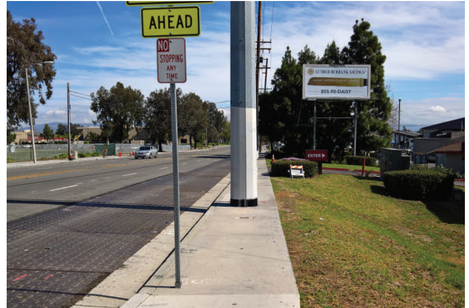
Obstructions in the sidewalk
