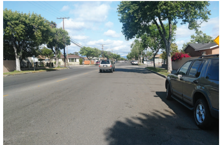
Excess right of way, missing crosswalks and bicycle routes
