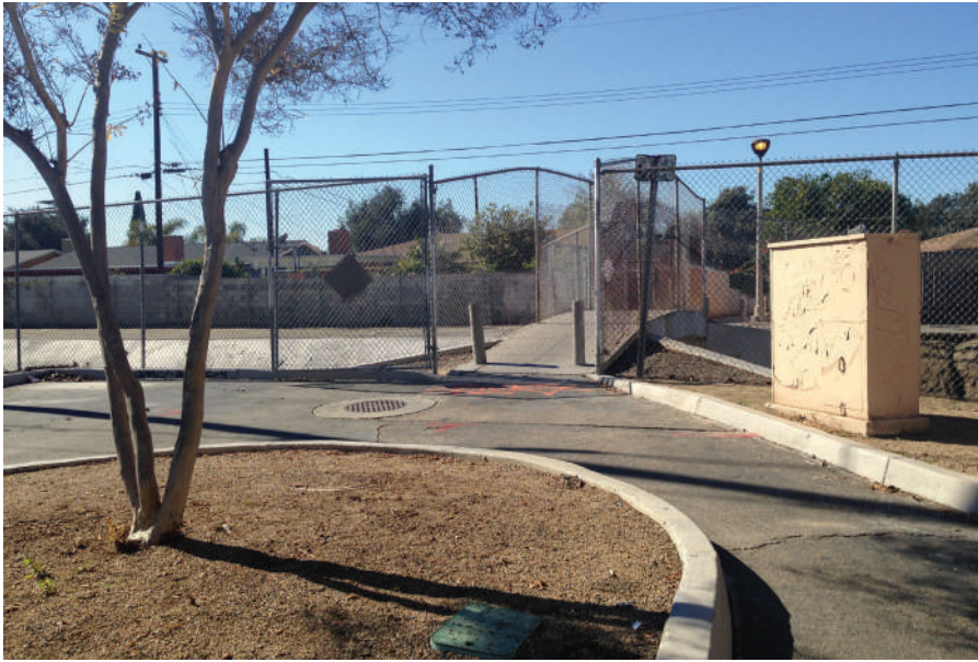
Pedestrian and bicycle bridge
