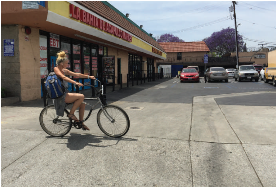
Missing sidewalks at Edinger Avenue
