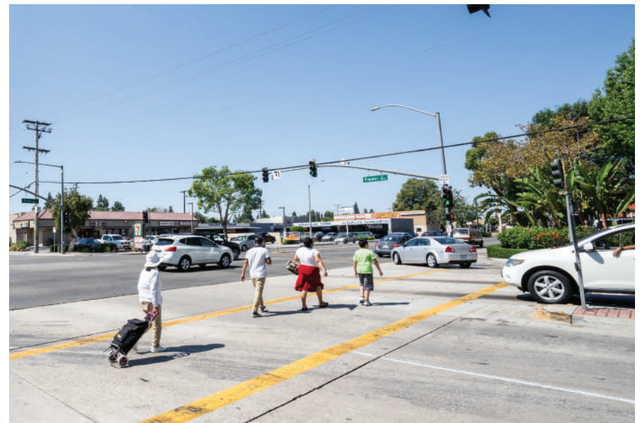
Improve traffic signal timing for pedestrians, lack of enhanced crosswalks
