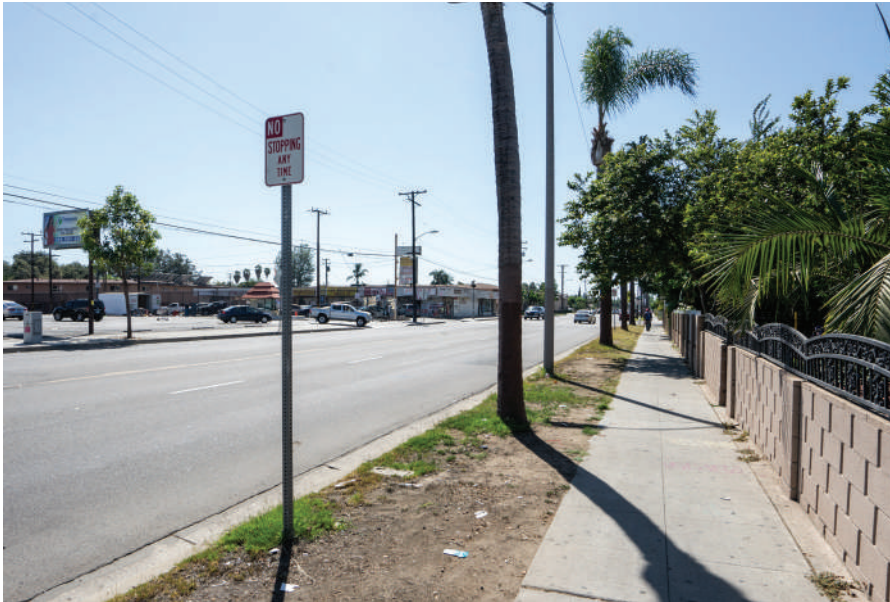
Narrow sidewalk and excess right of way
