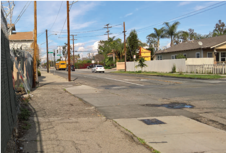
Missing sidewalk and excess right of way
