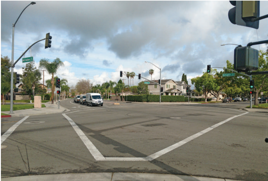
Lack of enhanced crosswalks
