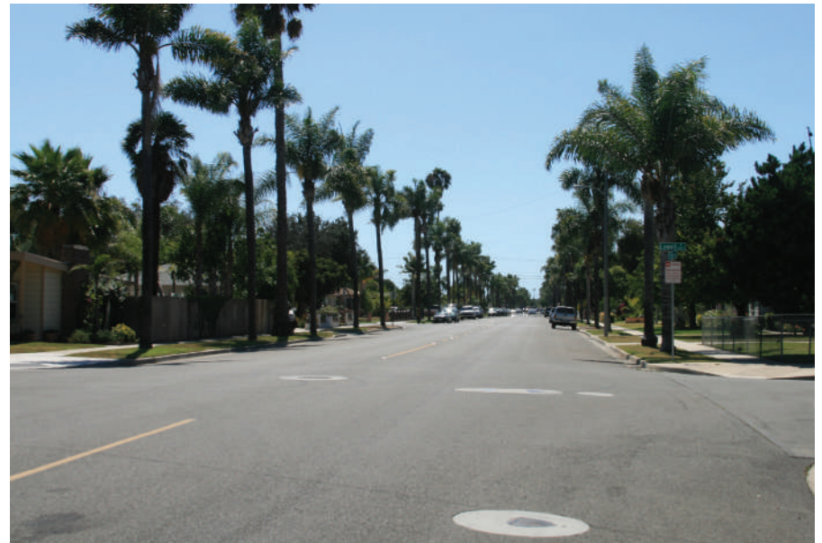
Lack of bicycle routes, excess right of way
