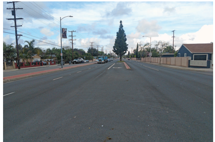
Multiple lanes and long blocks without crossings
