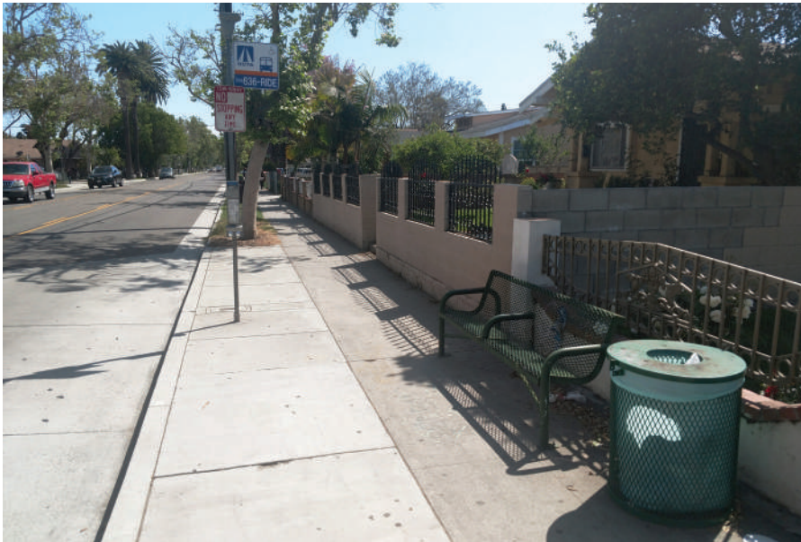
Bus stop with no shelter
