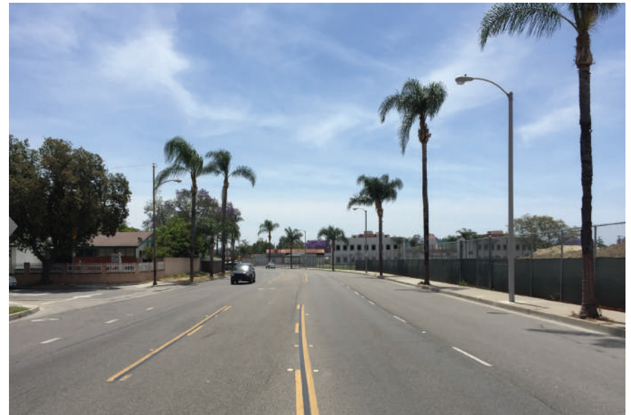
Multi-lane road with segments without parkways for additional pedestrian separation adjacent to a school.
