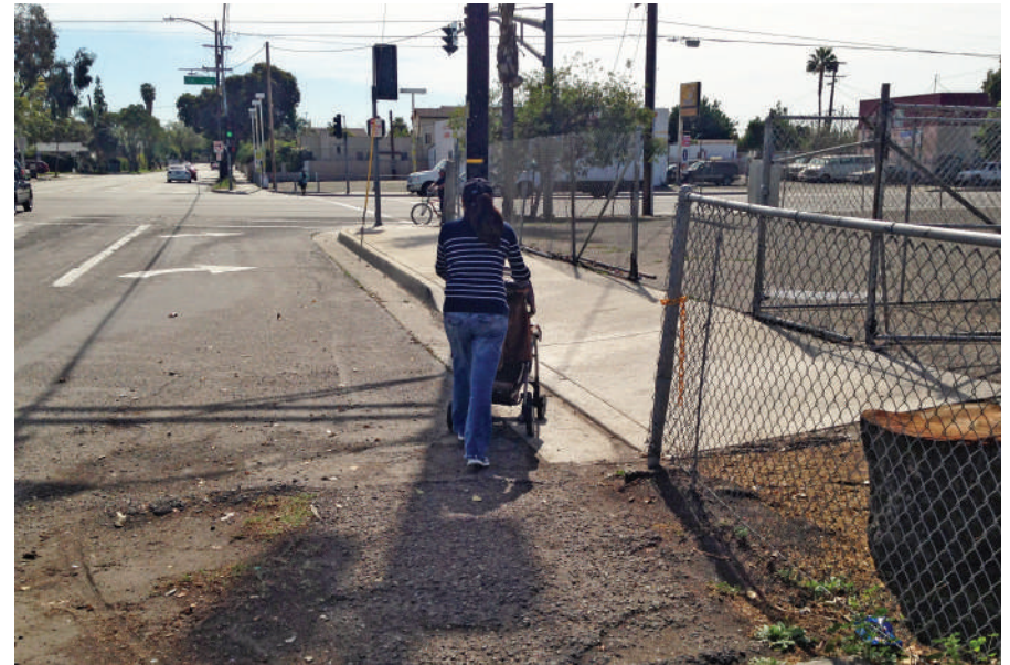
Missing sidewalk and excess right of way
