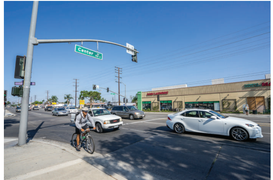
Missing sidewalk and excess right of way
