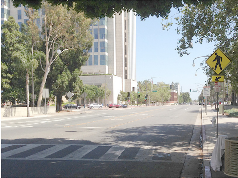
Enhanced crosswalk with pedestrian flashers at City Hall
