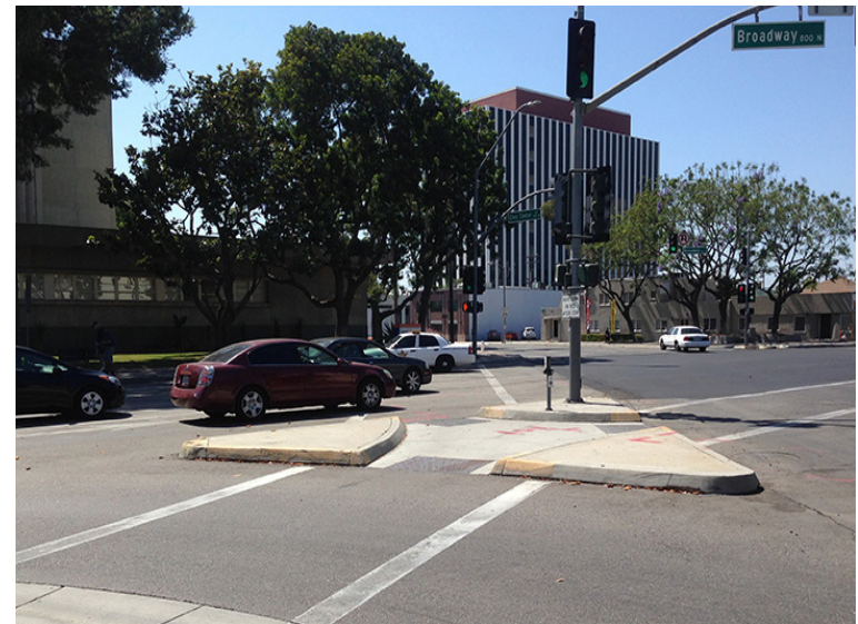
Pedestrian refuge for two-phased crossing at Broadway
