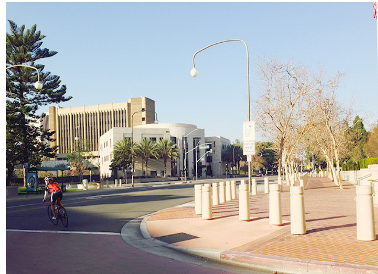
Curb extensions and decorative paving in crosswalk at Fourth Street
