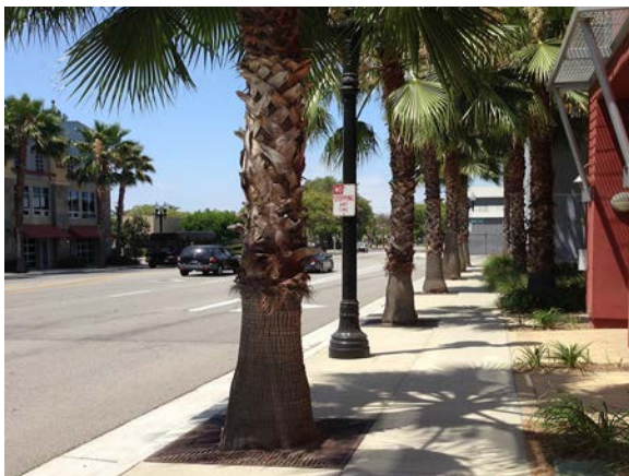
High traffic volume streets adjacent to sidewalks (Santa Ana Boulevard)
