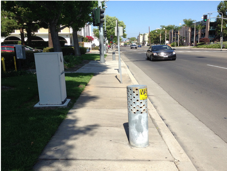
Lack of pedestrian buffers from travel lanes
