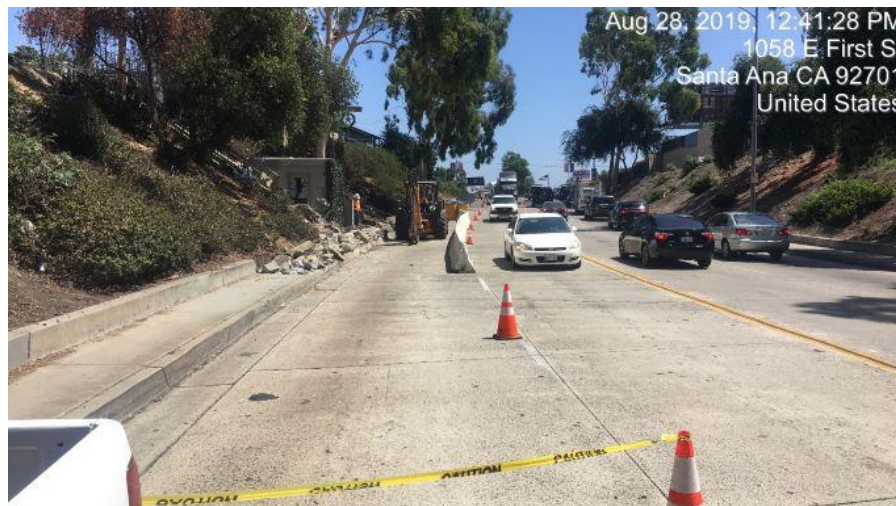
First Street Lift Station
