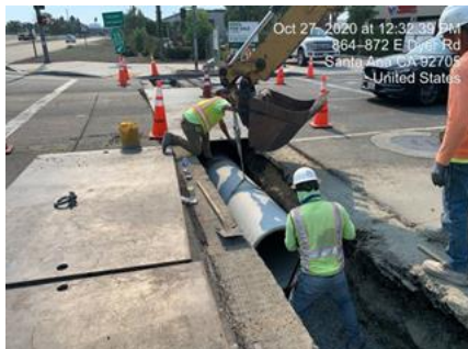
Dyer Road Stormdrain Repair
