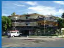
Sixth Street Rehabilitation
