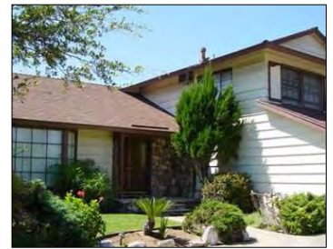
Community Care facility
