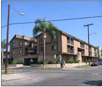
The Redevelopment Agency funded the rehabilitation and reconfiguration of the Ross Durant Apartments, adding long-term affordability covenants.
