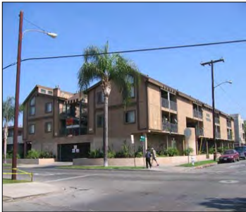
The City funded the rehabilitation and reconfiguration of the Ross Durant Apartments, adding long-term affordability covenants.
