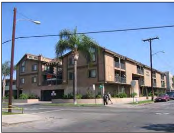
Recent Acquisition and Rehabilitation Project
