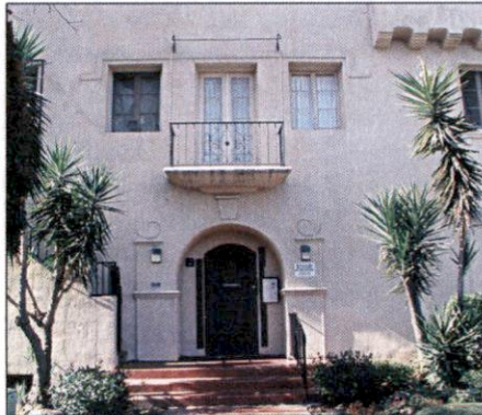
Illustrative Photo: Stacked Dwellings with a stoop entry
