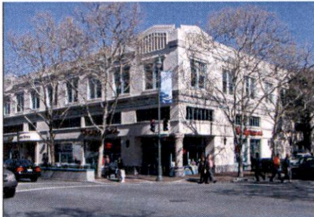
Illustrative Photo: Flex Block with shopfront frontage
