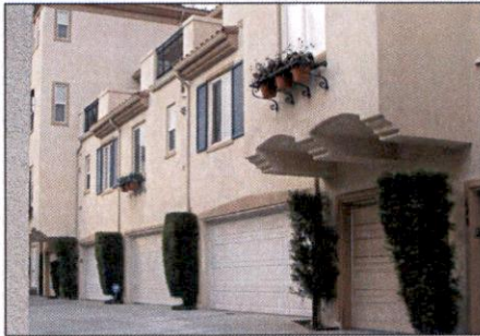
Illustrative Photo: Tuck-under garage access
