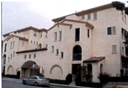
Illustrative Photo: Architecture of two individual tuck-under buildings combined at the alley access that separates the two buildings
