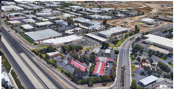
BEFORE 55 FREEWAY AND DYER ROAD
