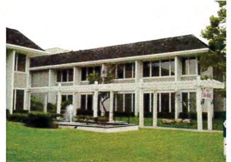
19 Fourth Street Looking Northwest from Intersection on Golden Circle Drive
