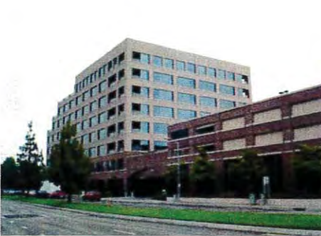
17 Fourth Street Looking South to Commercial Building
