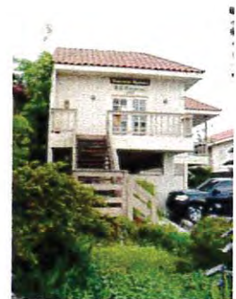
44 Tustin Avenue West Side
