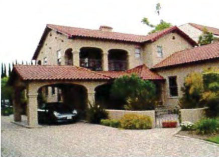
43 Tustin Avenue West Side
