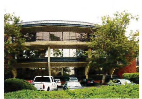
25 The Theme Building from the Southwest
