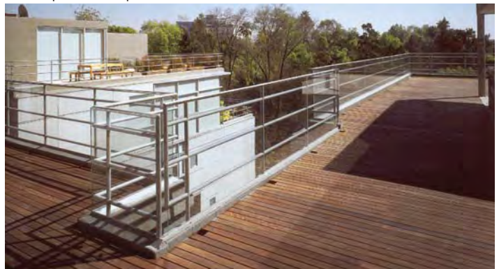
Private rooftop deck
