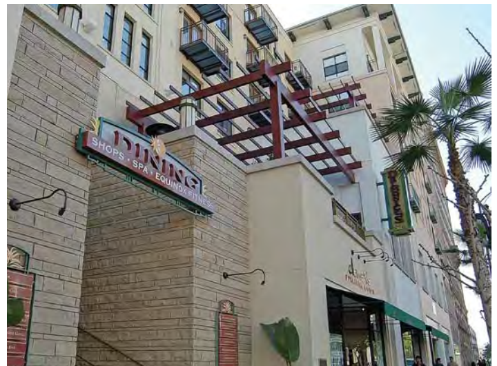
Street-facing facade elements
