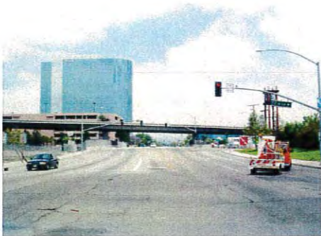
4 First Street View East
