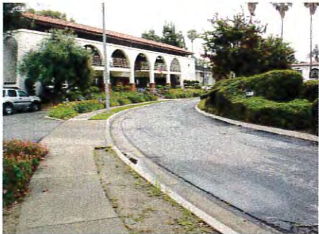
26 Golden Circle Drive: Western Section Looking North
