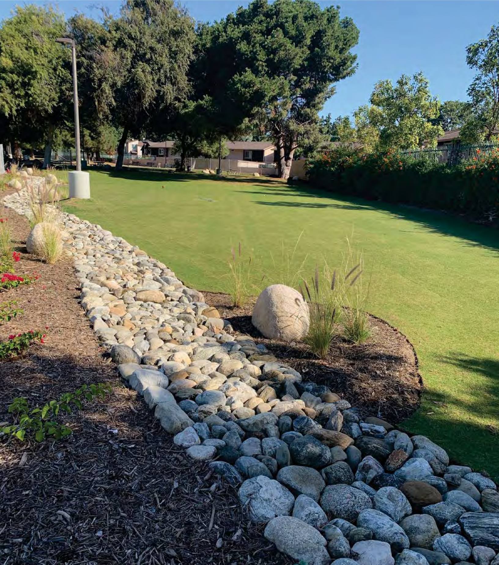
Mabury Park Stormwater Project. Completed in 2019, the project included the construction of a 7,000-square-foot bioretention basin designed to capture and infiltrate approximately 27,000 cubic feet of stormwater during a significant storm. The bioretention basin will capture stormwater runoff and use natural filtering through the soil to remove pollutants before it is released into the City's storm drain system. This project was the first regional stormwater infiltration best management practice (aka BMP) in the City of Santa Ana.
