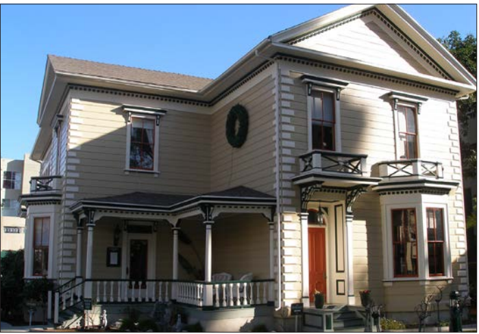
Illustrative Photo: Duplex with Porch Frontage
