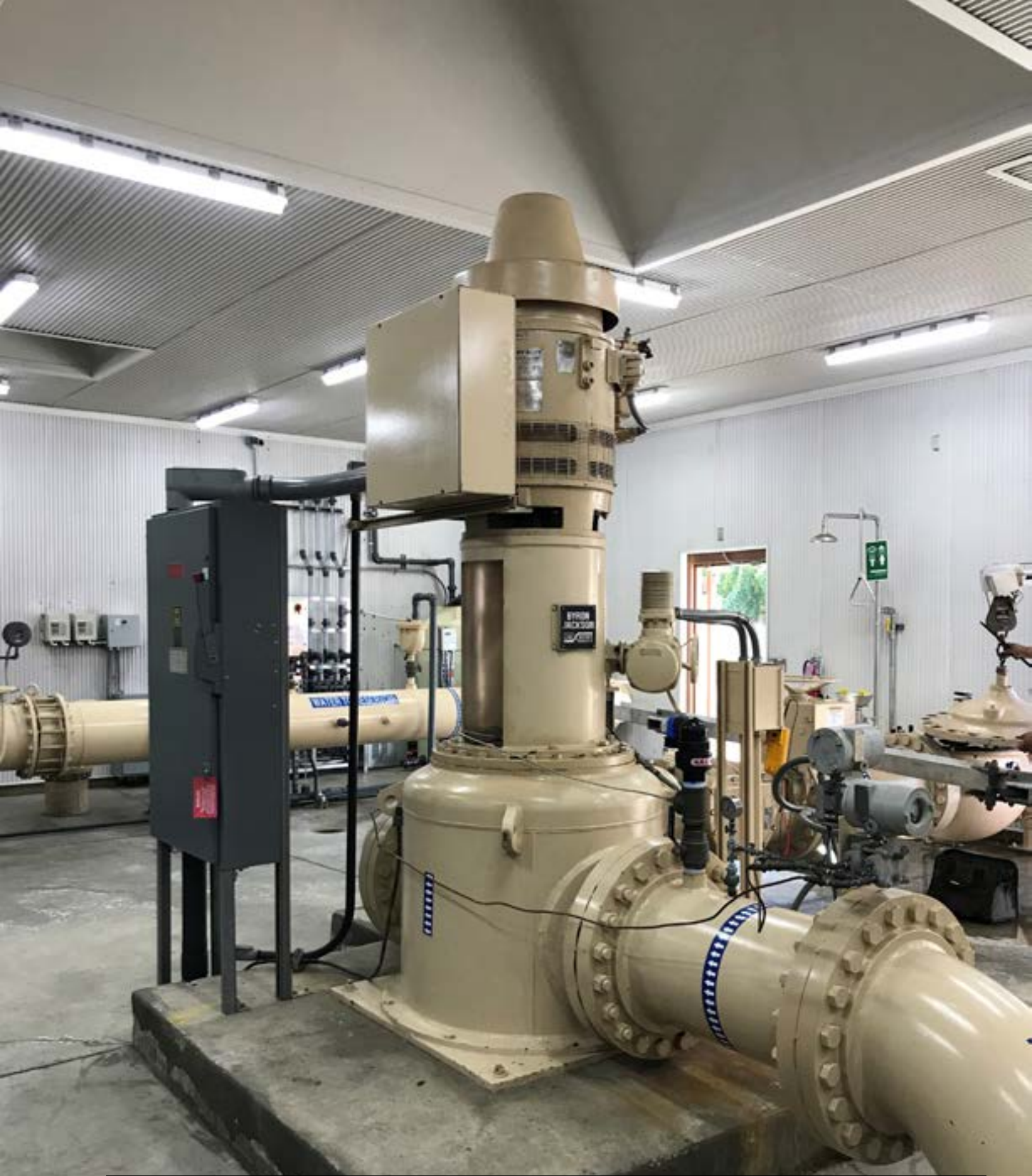
Hydropower: The City's Public Works Agency purchases millions of kilowatt-hours every year to operate well pumps and booster pumps to deliver clean water. The City continuously evaluates and implements onsite renewable energy systems (shown here is a hydropower project) to offset some of this electric load, lowering electric bills and reducing the associated greenhouse gas emissions.
