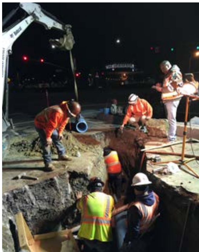
▲ Maintaining utility systems 24-7 [cover photo]
