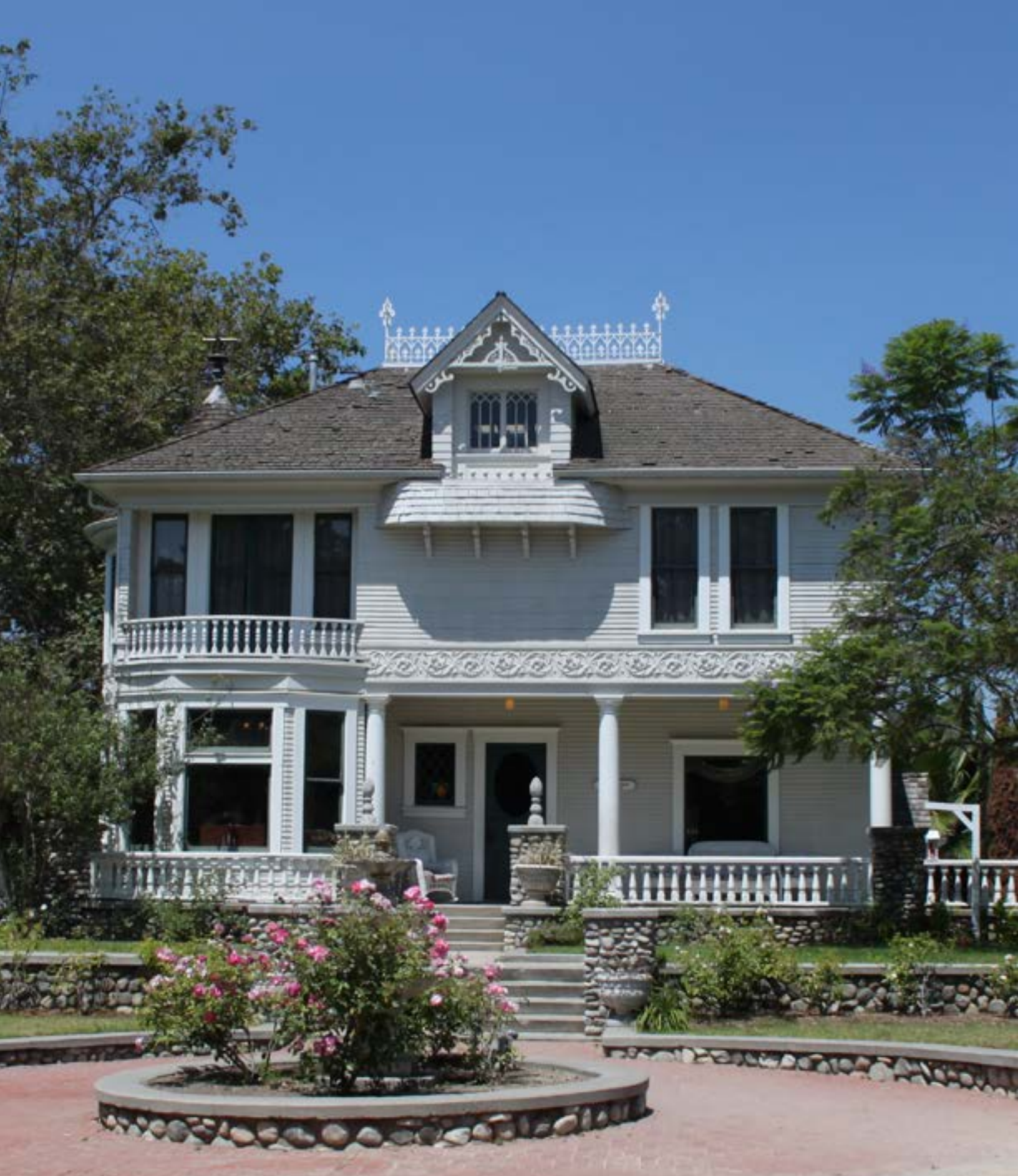
The Kellogg House. With its asymmetrical shape, faux tower, and prominently decorated dormer, the Kellogg House is a late example of Queen Anne—style Victorian architecture. The house was originally located in downtown Santa Ana at 122 Orange Street. It was donated to the Heritage Museum of Orange County and moved to the museum's grounds in 1980. Today, it provides hands-on opportunities to educate visitors about the Victorian era.
