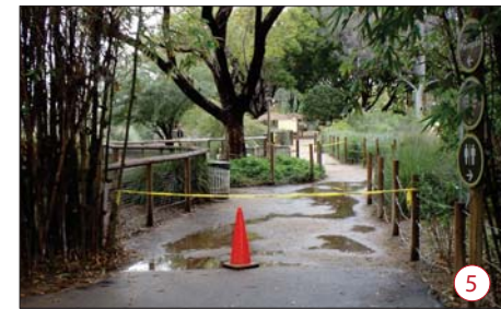
ERODED DIRT PATHS
