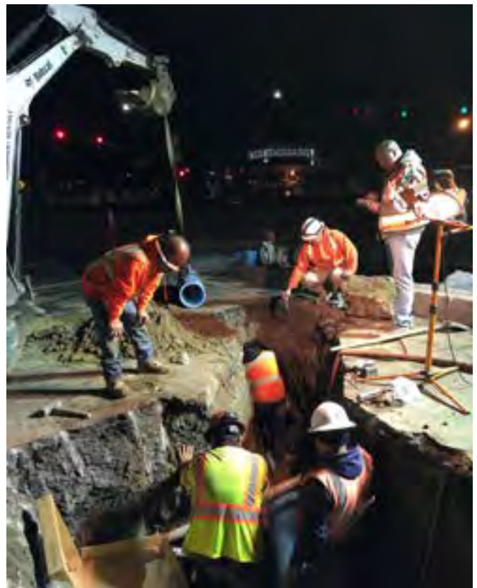
▲ Maintaining utility systems 24-7 [cover photo]
