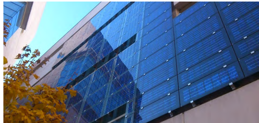
Green roofs and solar panels are two methods to reduce energy costs through building design.
