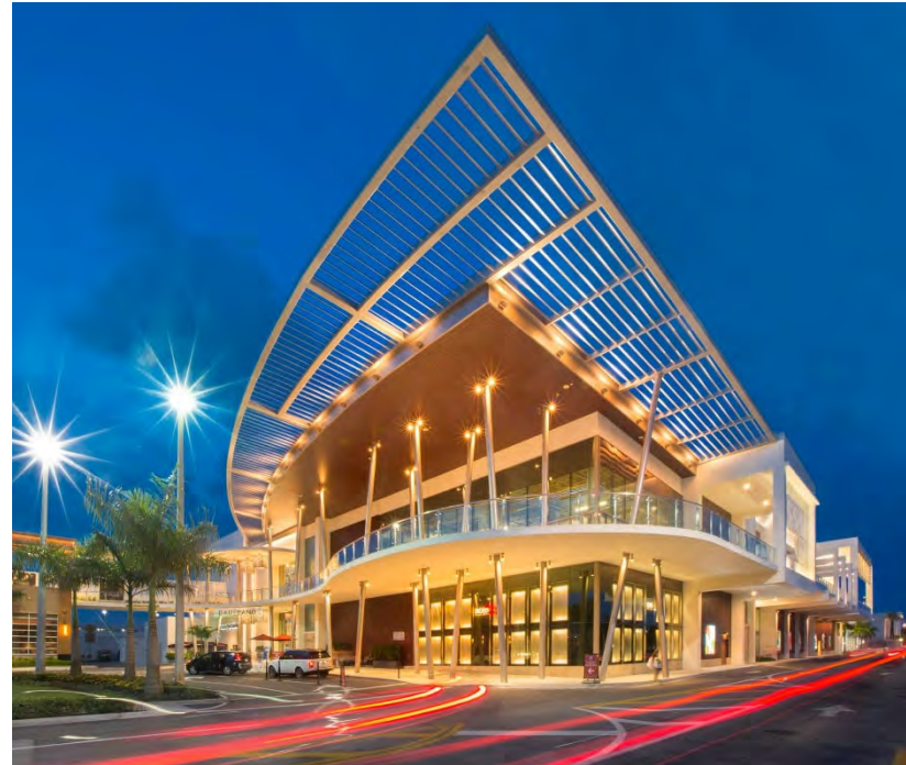
Building lighting at the pedestrian level creates inviting spaces at night.
