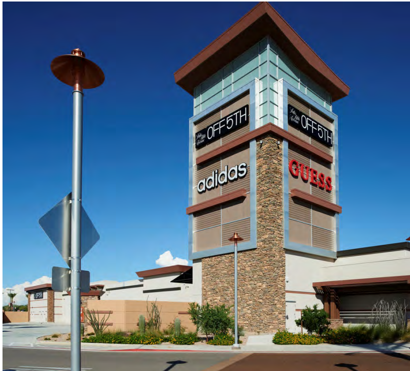
Signage for multiple tenants or businesses should be consolidated and designed to be cohesive.
