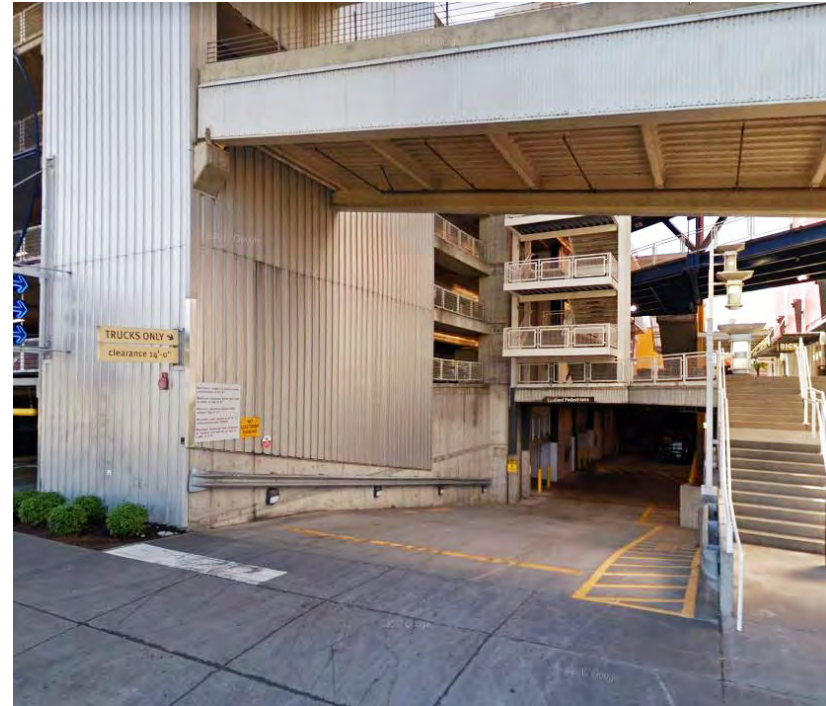
An example of one method used to hide the service facilities for a big-box retail store.
