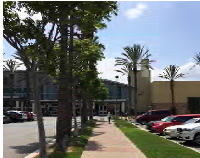
A dedicated pedestrian walkway through a parking lot to increase pedestrian safety.
