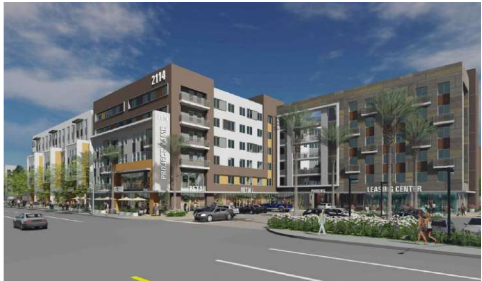
AMG & Associates is building a 552-unit affordable family project in Santa Ana
