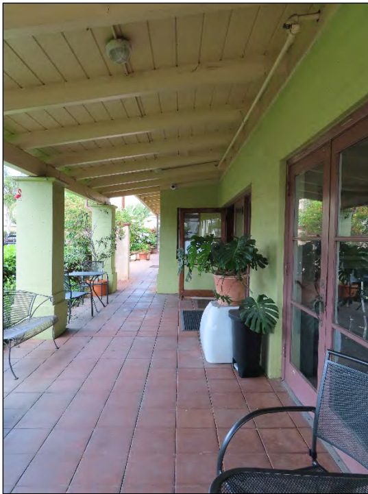
View east of the main (north) entrance porch.
