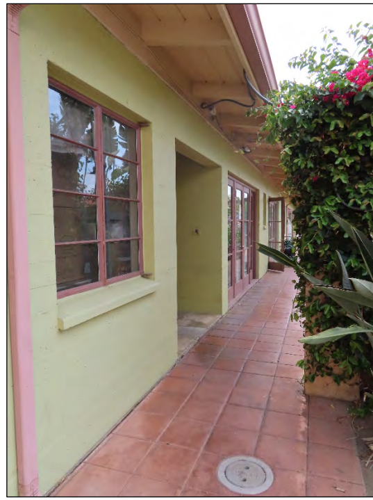
View west of the north façade.
