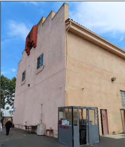
View southeast of the north façade.
