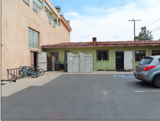
View south of the north façade of the east-west wing and west façade of the north-south wing.
