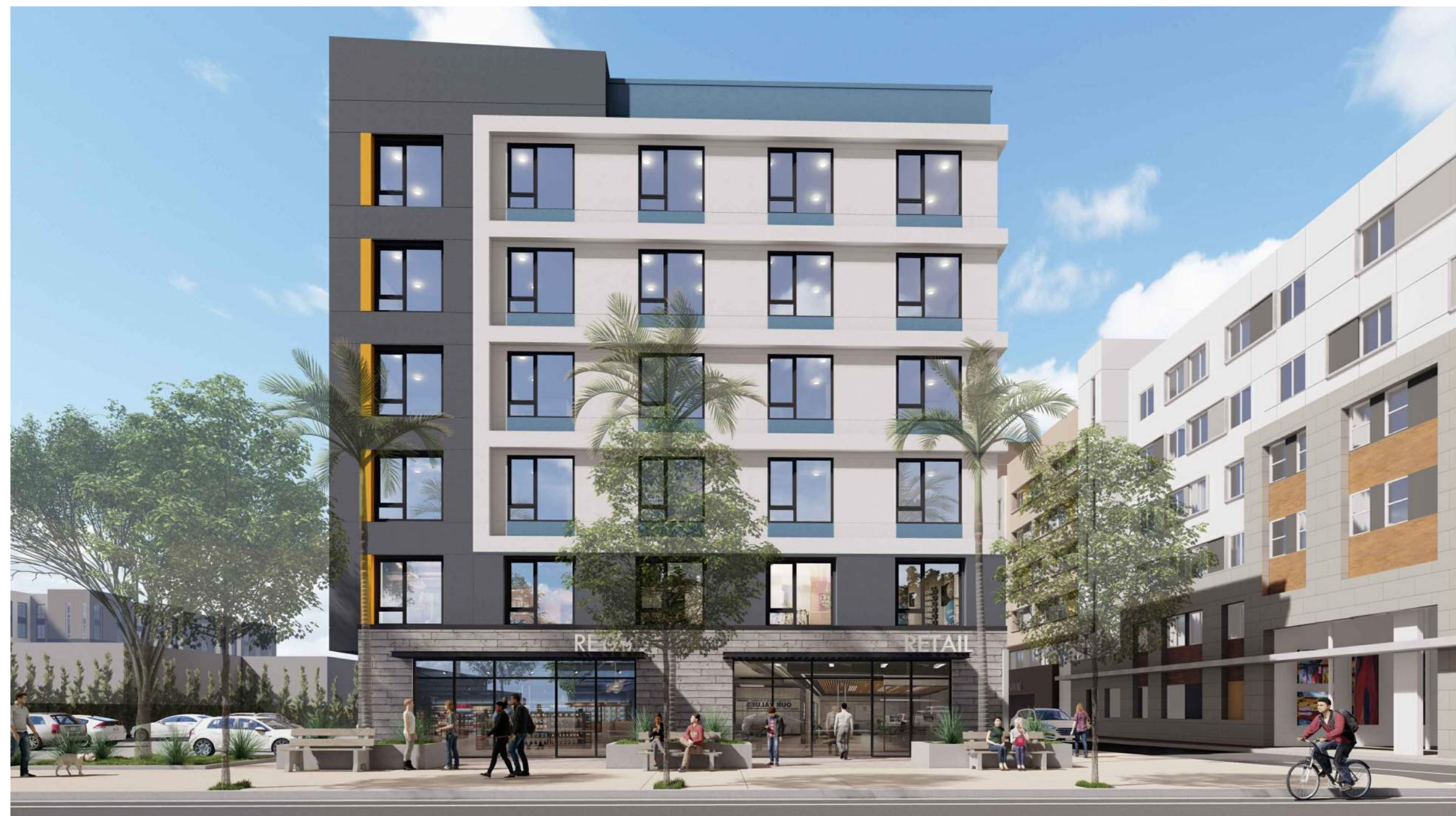
VIEW ON FIRST STREET LOOKING SOUTH 3
