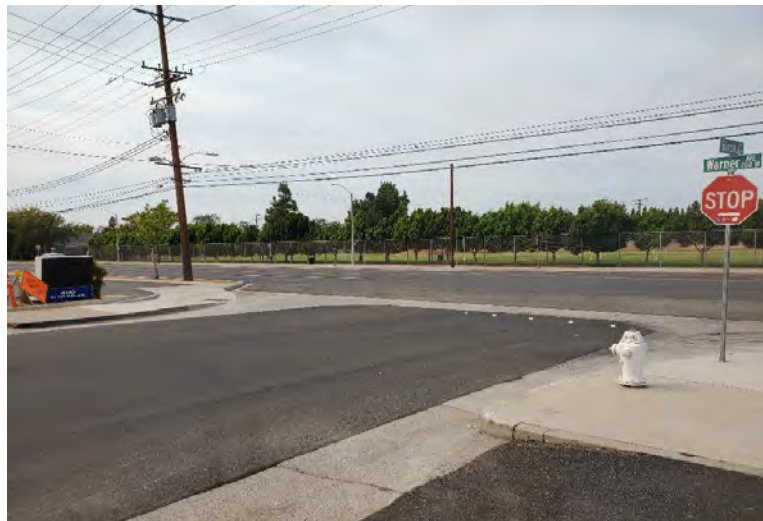
Garnsey Business District Pavement Rehabilitation
