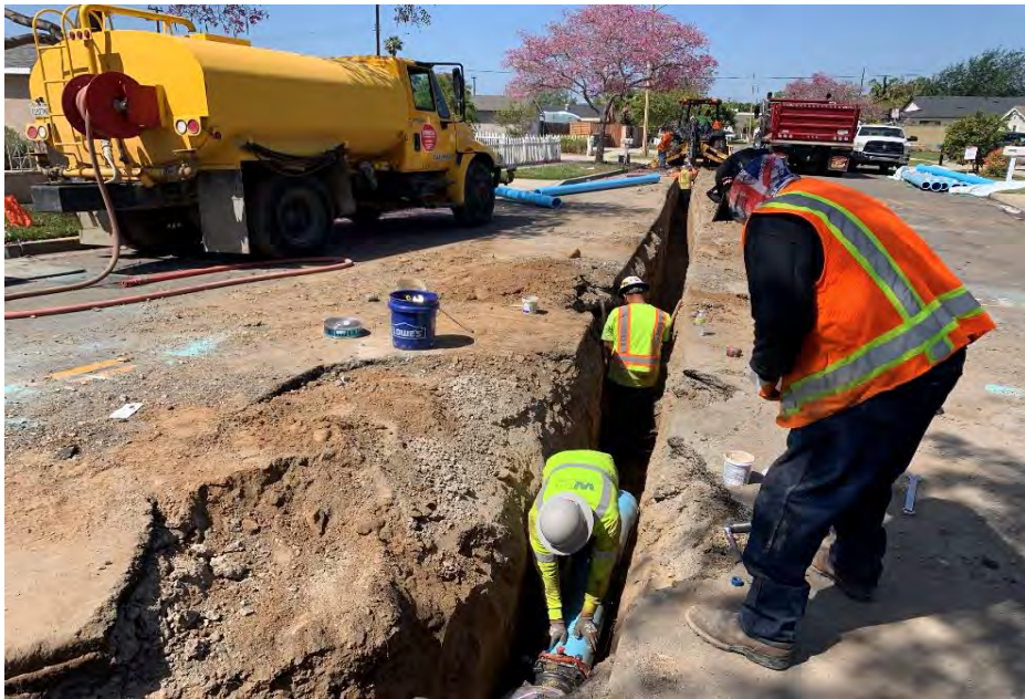
Grovemont Water Main
