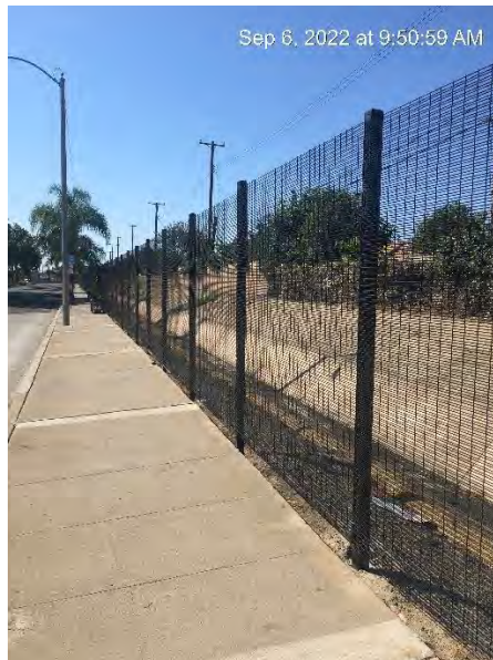
Stormwater Channel Fencing Upgrades
