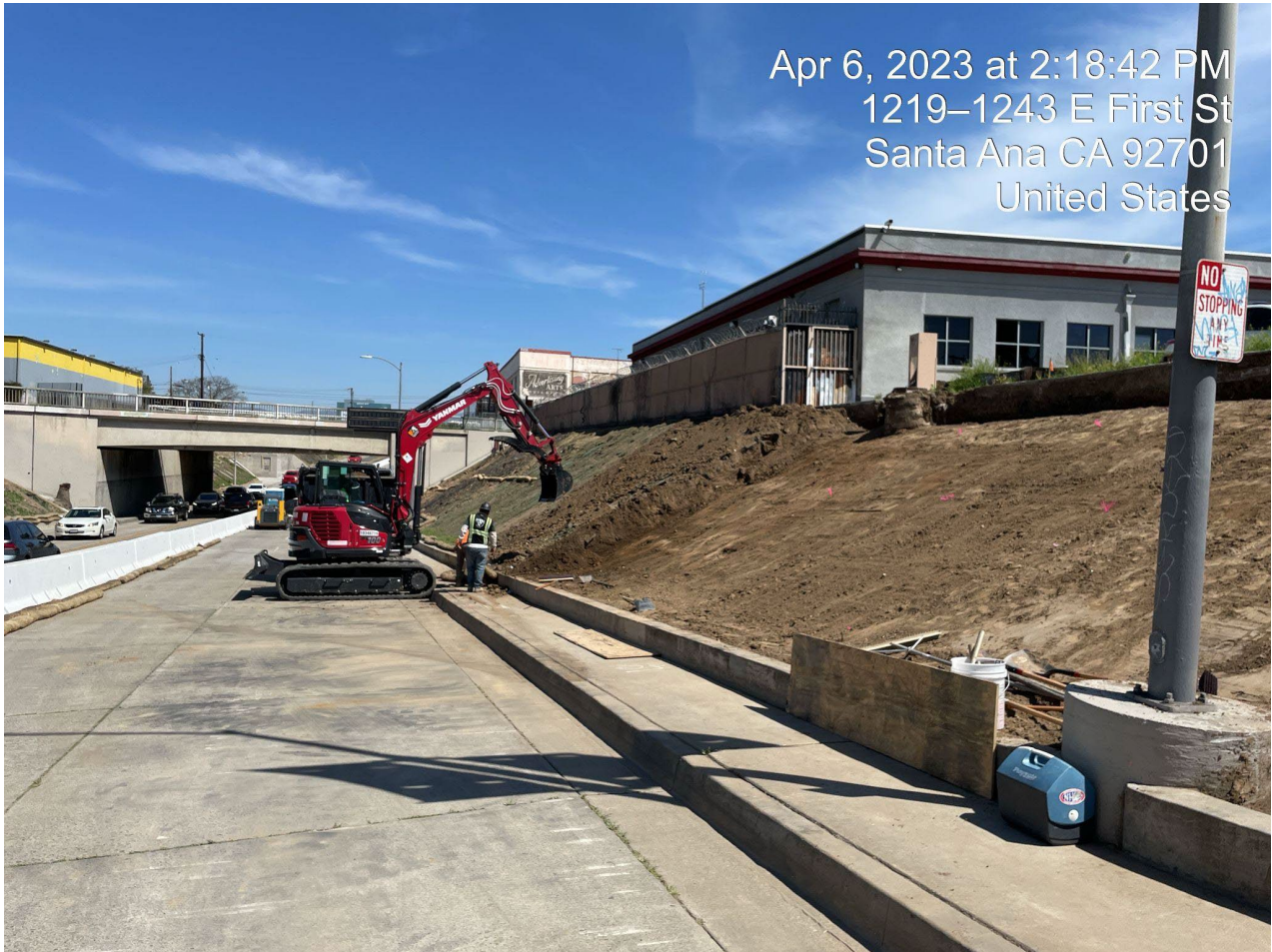
Grading of dirt slopes
