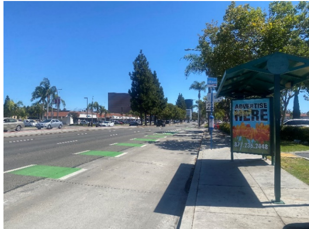
Bristol Street Existing Condition
