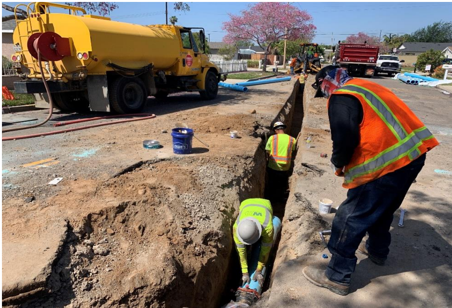
Grovemont Water Main
