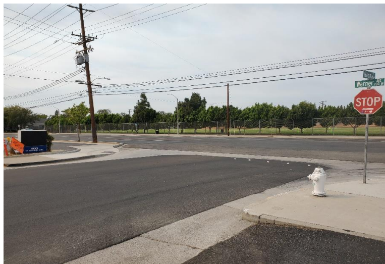
Garnsey Business District Pavement Rehabilitation
