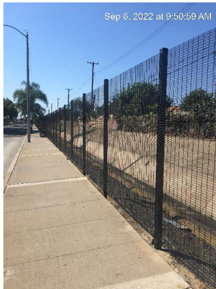
Stormwater Channel Fencing Upgrades
