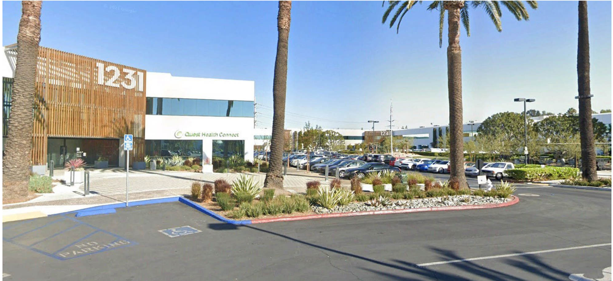
View of 1231 Dyer Road from Tech Center Drive
