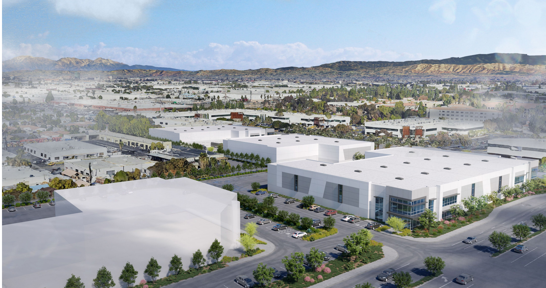
Aerial view from Dyer Road Looking East toward project site
