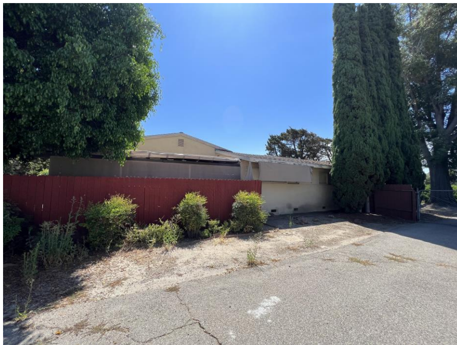
Photograph 8. North end of the west elevation, facing southwest.
