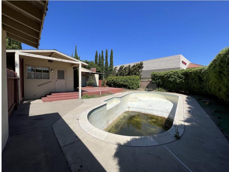
Photograph 6. Overview of east elevation and backyard area, facing northwest.
