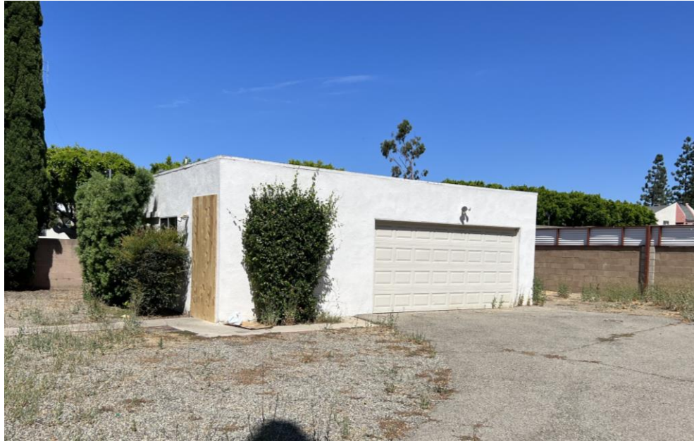
Photograph 8. Overview of detached garage, facing northwest.
