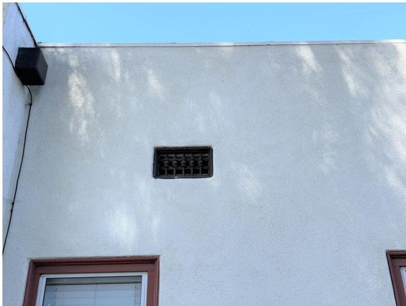
Photograph 3. Detailed view of vents over windows, facing west.
