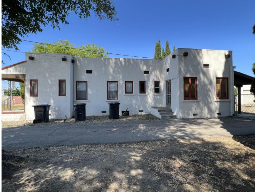
Photograph 2. Overview of east elevation, facing west.
