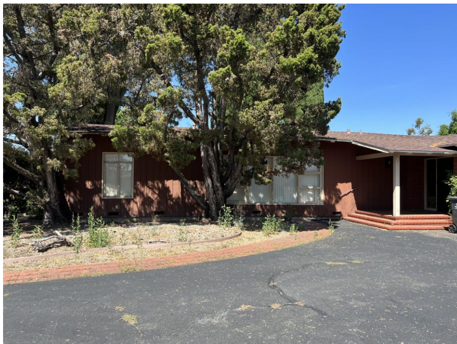
Photograph 3. Overview of front portion of east elevation, facing west.
