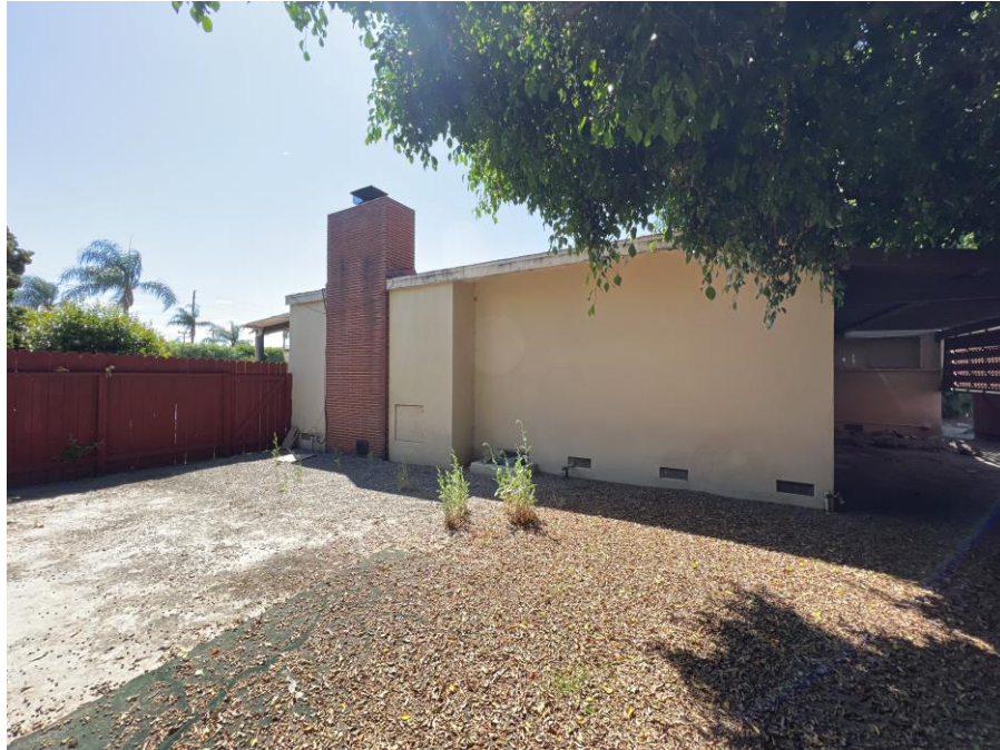
Photograph 10. Chimney on north elevation, facing southeast.
