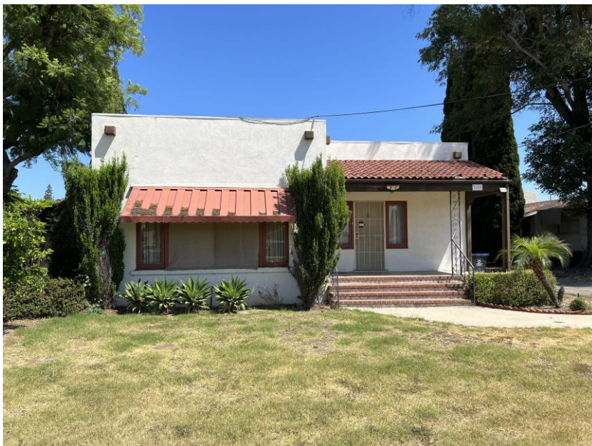
Photograph 1. Overview of primary (south) elevation, facing north.
