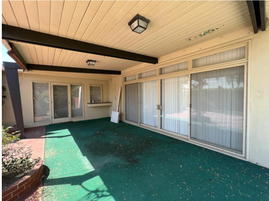
Photograph 4. Detailed view of covered patio area, facing southwest.
