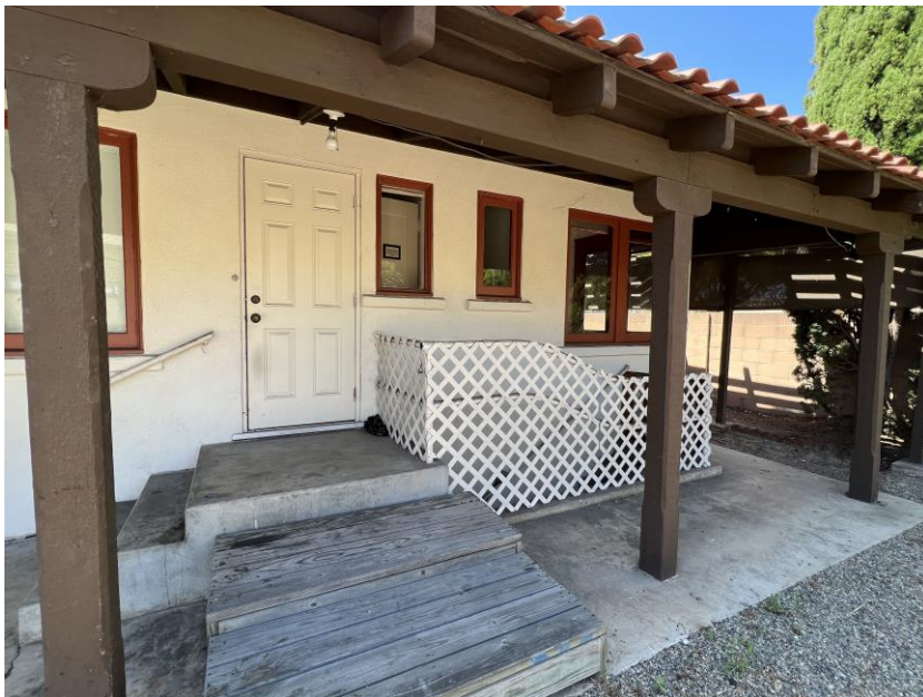
Photograph 5. Detailed view of the staircases on the north elevation, facing southwest.
