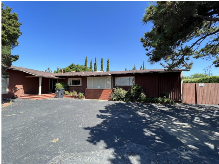
Photograph 1. Overview of primary (south) elevation, facing northwest.
