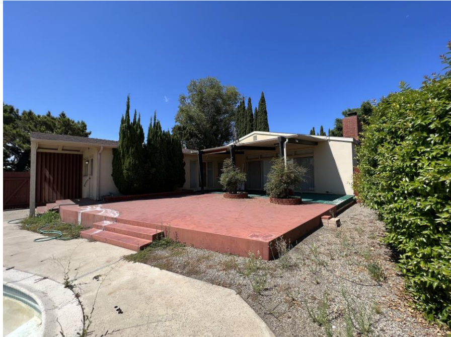
Photograph 5. Overview of rear portion of east elevation, facing southwest.
