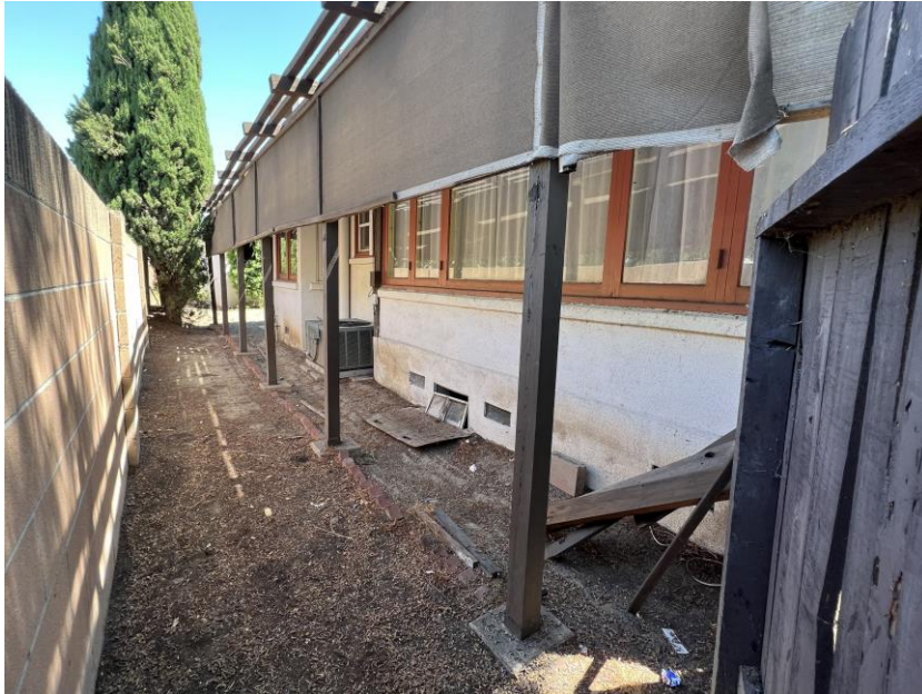
Photograph 6. Overview of north end of west elevation, facing northeast.
