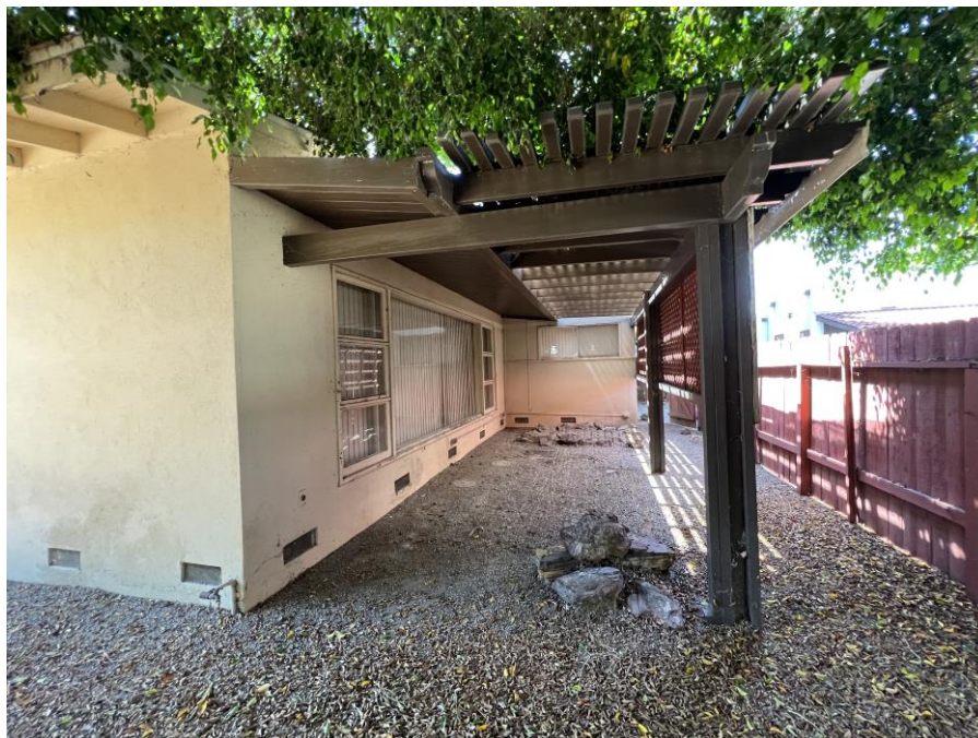
Photograph 9. Pergola area at northwest corner of the house, facing south.
