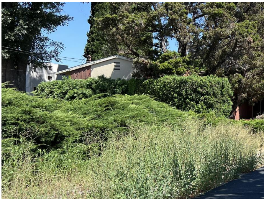
Photograph 2. Overview of southernmost point of south elevation, facing northwest.
