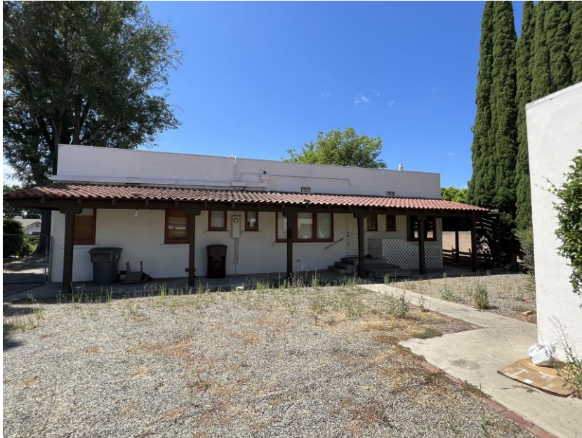
Photograph 4. Overview of north elevation, facing southwest.
