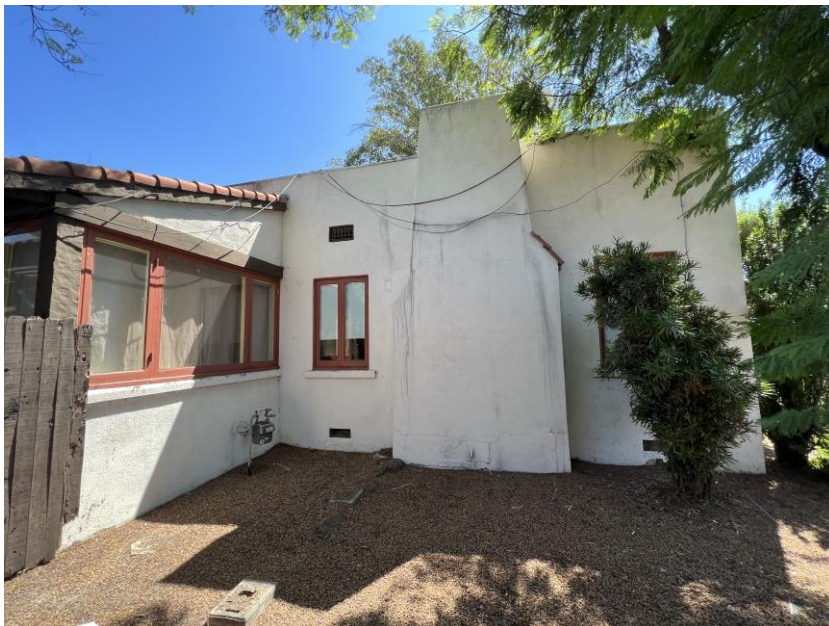
Photograph 7. Overview of south end of west elevation, facing east.
